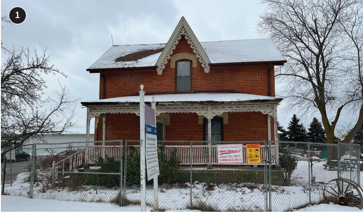
1 East elevation (ERA, 2024).
