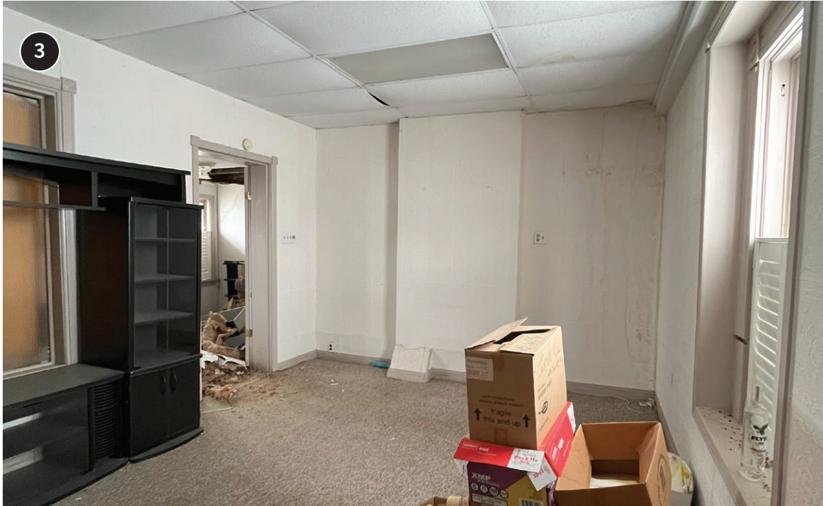
Interior, ground floor rear wing (ERA, 2024).
