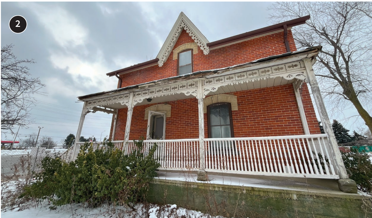
2 East elevation (ERA, 2024).
