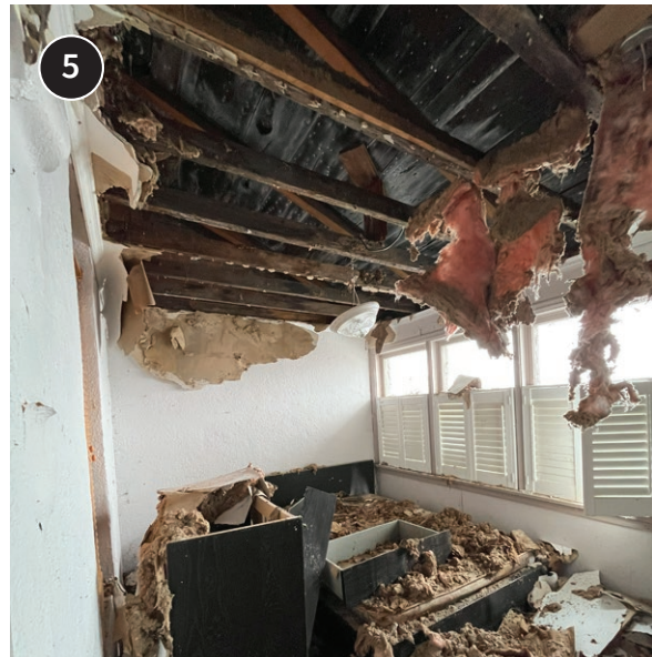
Interior, ground floor rear addition (ERA, 2024).
