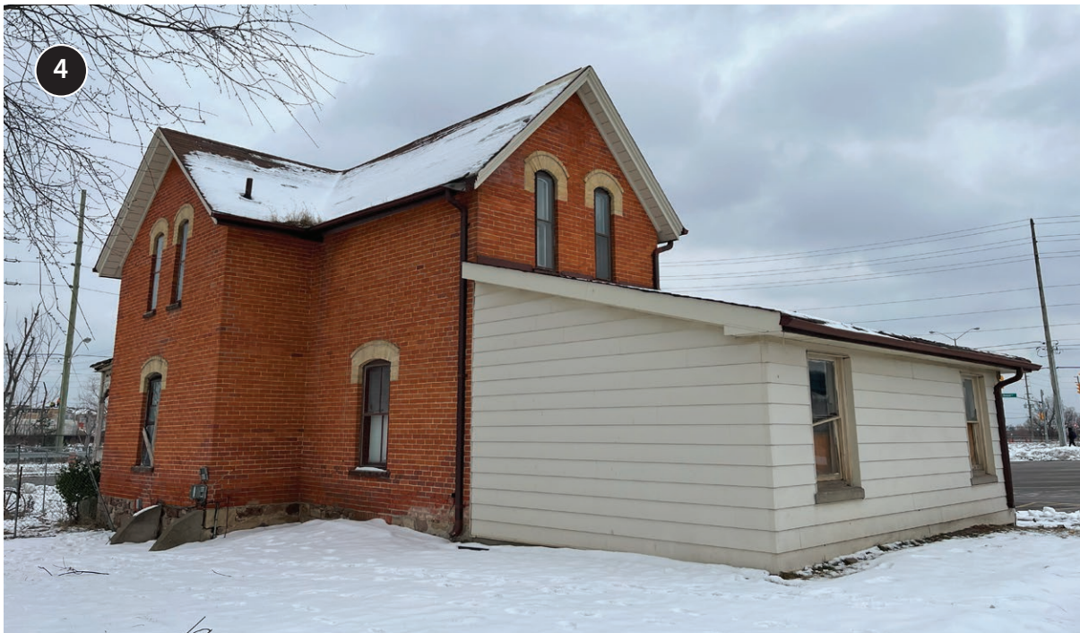
North and west elevations (ERA, 2024).
