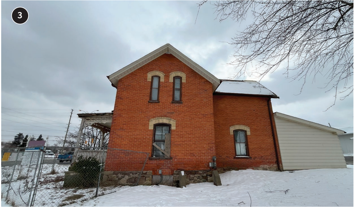
North elevation (ERA, 2024).
