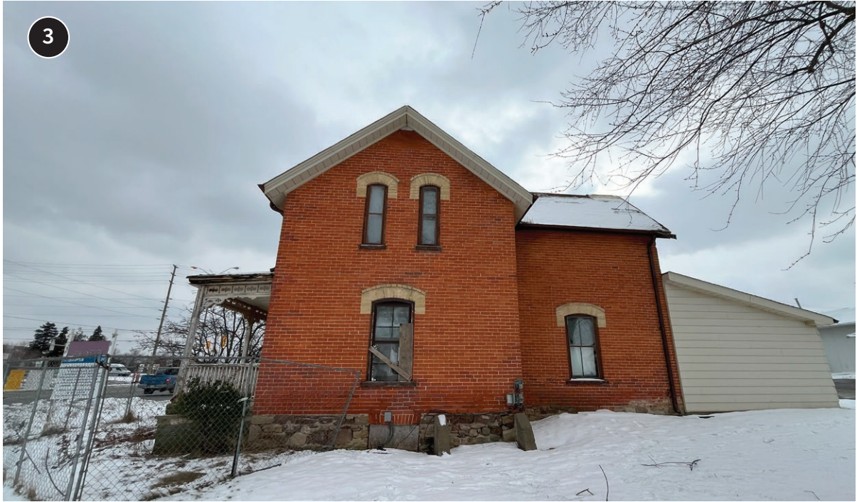
North elevation (ERA, 2024).
