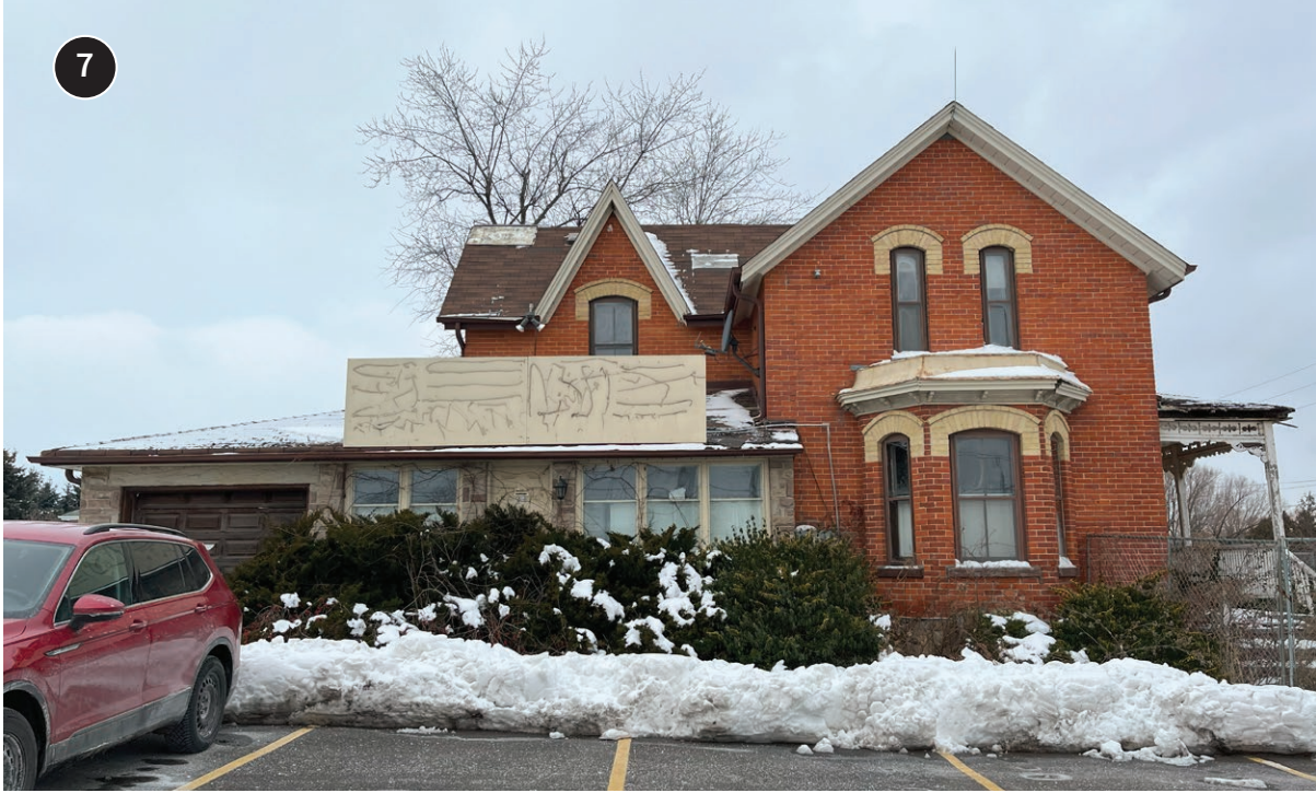
South elevation (ERA, 2024).
