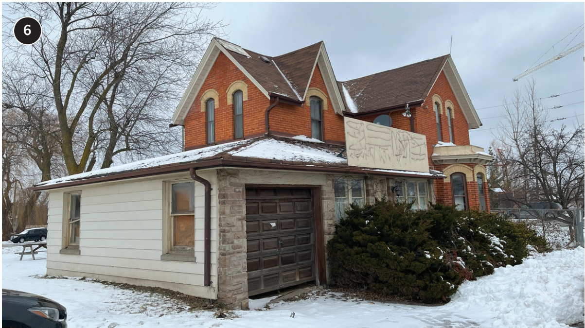
West and south elevations (ERA, 2024).
