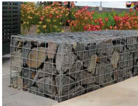
Decorative wall incorporating salvaged stones.
