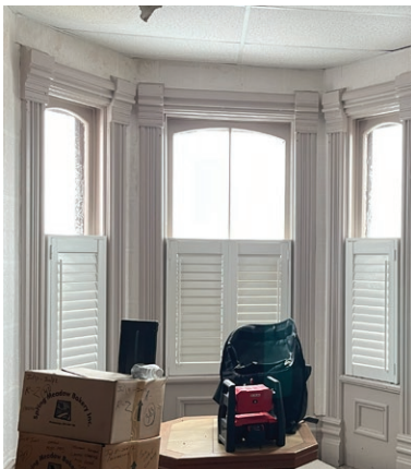
Interior wood trim (ERA, 2024).
