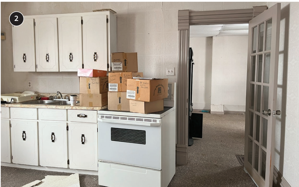
Interior, ground floor (ERA, 2024).
