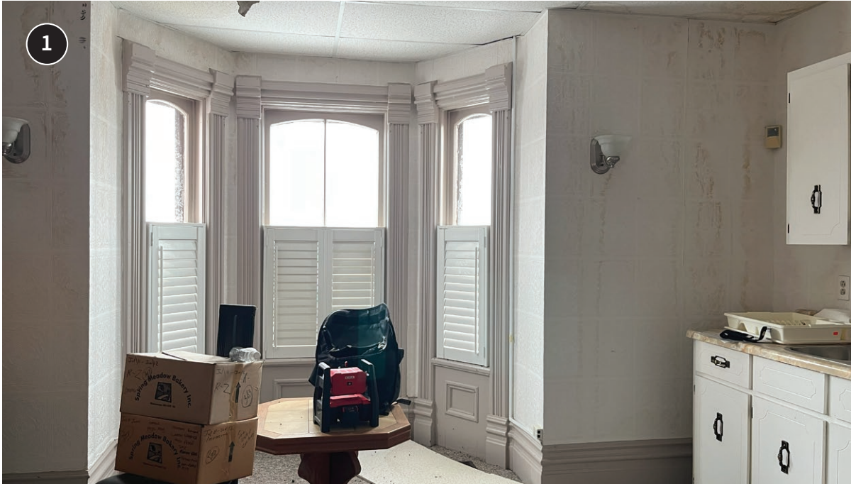
Interior, ground floor (ERA, 2024).
