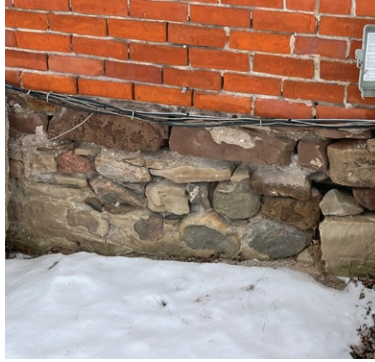
Fieldstone foundation (ERA, 2024).
