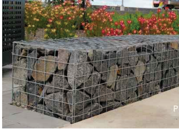
Decorative wall incorporating salvaged foundation stones.
