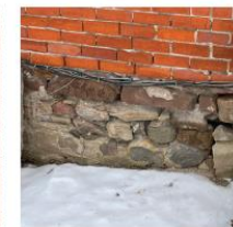
Fieldstone foundation (ERA, 2024).
