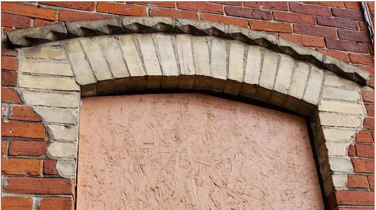
Image 15. View northeast showing a typical buff brick voussoir on a window on the first storey of the southwest elevation of the house on the Property
