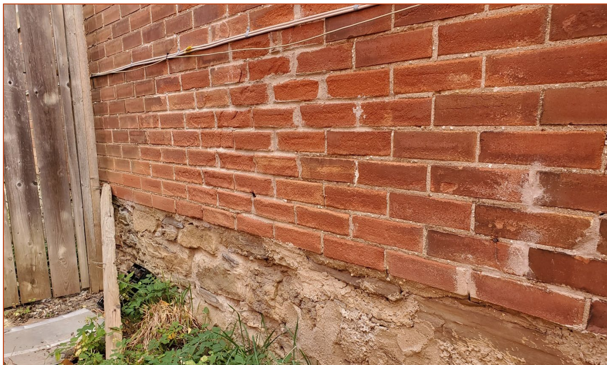
Image 13. View north showing the stone foundation and brick on the first storey of the southwest elevation of the house on the Property
