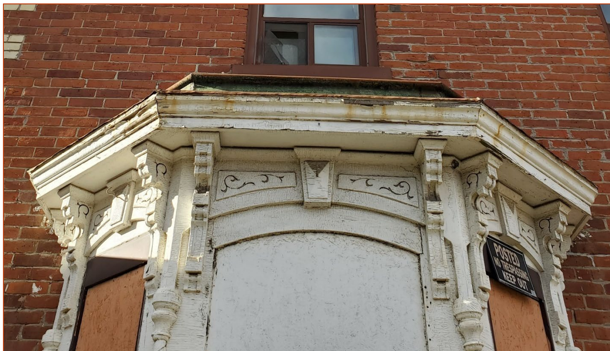
Image 20. View southwest showing the roof structure and wooden frame of the bay window on the northeast elevation of the house on the Property
