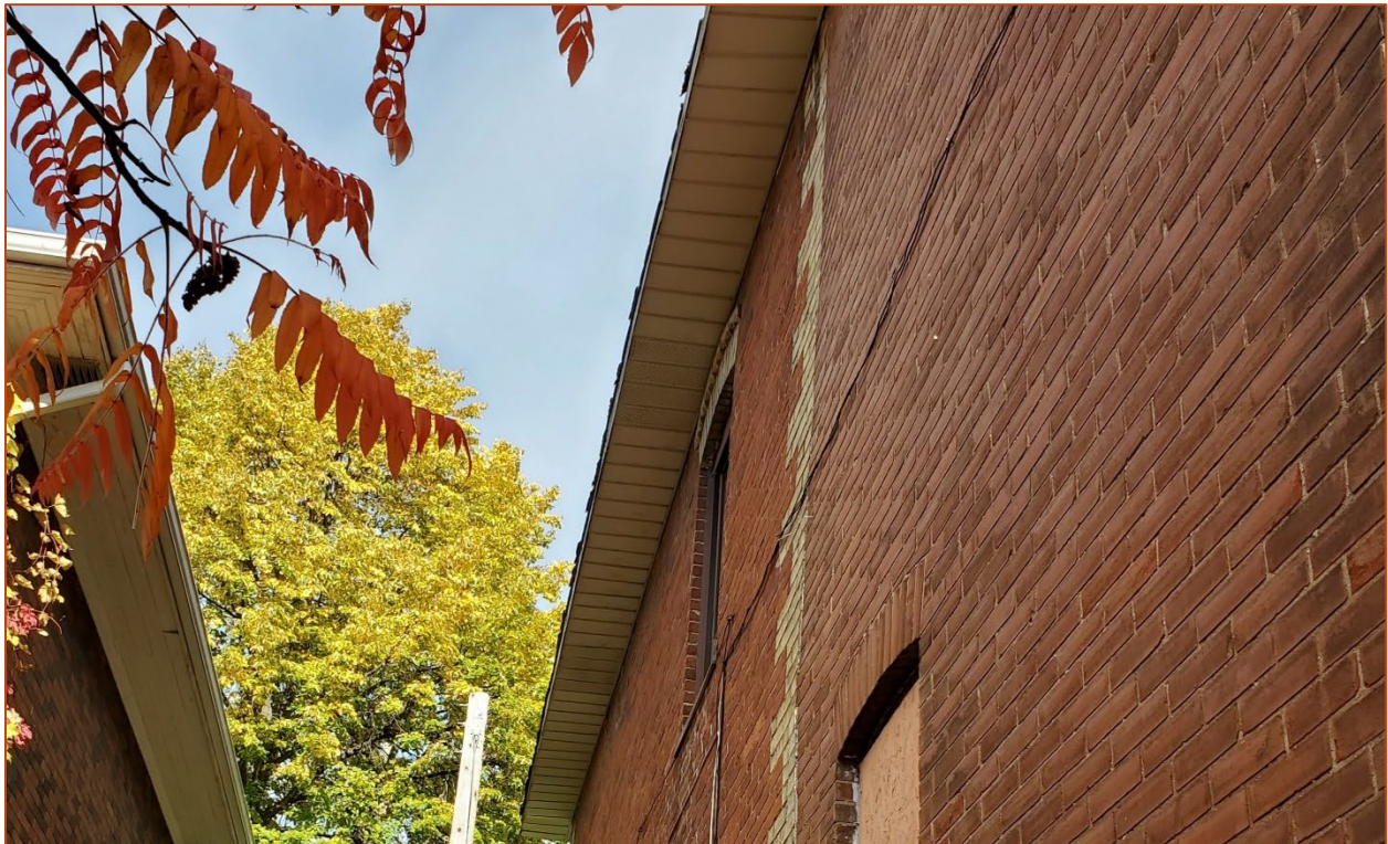
Image 27. View north showing the projecting eave and soffit of the roof on the southwest elevation of the house on the Property
