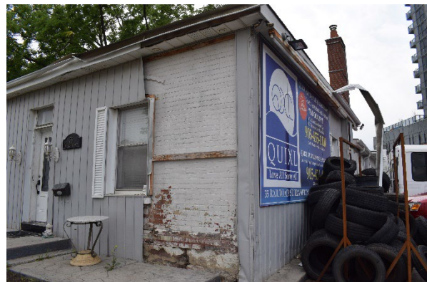
Photo 4.20: 35 Railroad Street original brick wall and stone foundation
