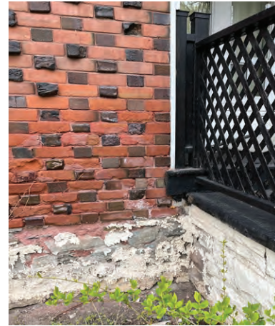
Close-up of clinker brick treatment at 43 Mill Street North (ERA, 2023).
