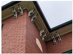
Image 25: Detail of paired brackets under the eaves.
