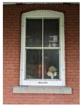
Image 21: View of a segmentally arched window on the farmhouse's front facade.
