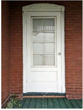
Image 24: View of one of the front doors, note the perforated design above the door and decorative wood surround.
