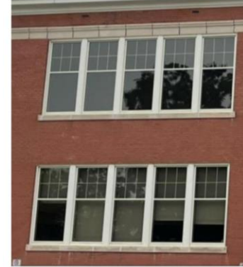
Photograph 16: View of the six-over-one, attached fixed pane windows on the south elevation (AECOM, August 2024)
