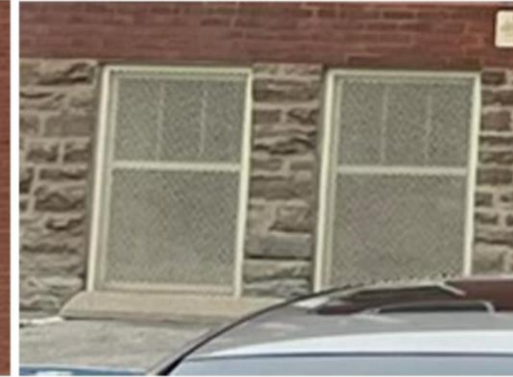
Photograph 18: View of the three-over-one, fixed-pane windows on the east elevation at the stone foundation (AECOM, August 2024)
