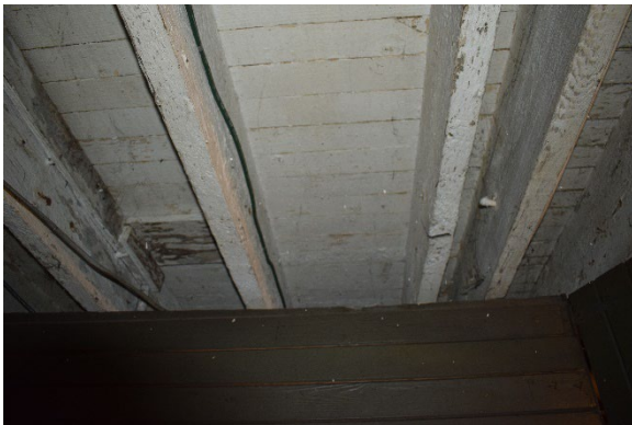
Plate 20 Basement interior, showing whitewashed floor joists
