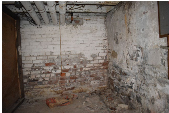
Plate 19 Basement interior, showing brick and stone foundations
