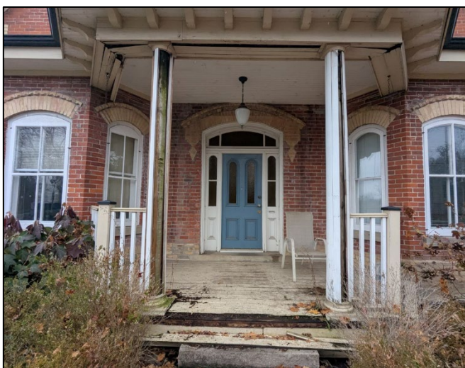
Figures 22-25: Views of incompatible cement repointing (top left), powdered bricks (top right), damaged and rotted portico wood (bottom left) and interior damaged plaster (bottom right). (MHBC, 2024)
