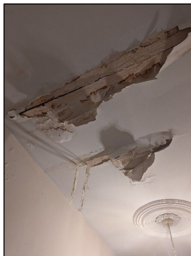
Figures 22-25: Views of incompatible cement repointing (top left), powdered bricks (top right), damaged and rotted portico wood (bottom left) and interior damaged plaster (bottom right). (MHBC, 2024)
