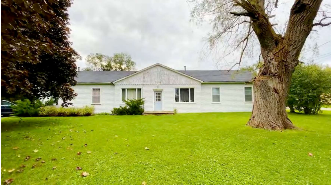
2305 Embleton Road – front elevation of 20 th century dwelling on the subject property that faces Embleton Road
