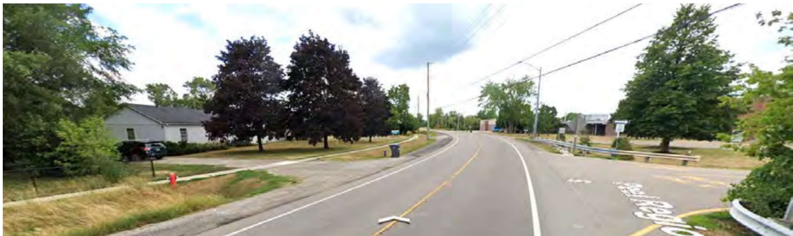
STREETVIEW – looking west along Embleton Road
