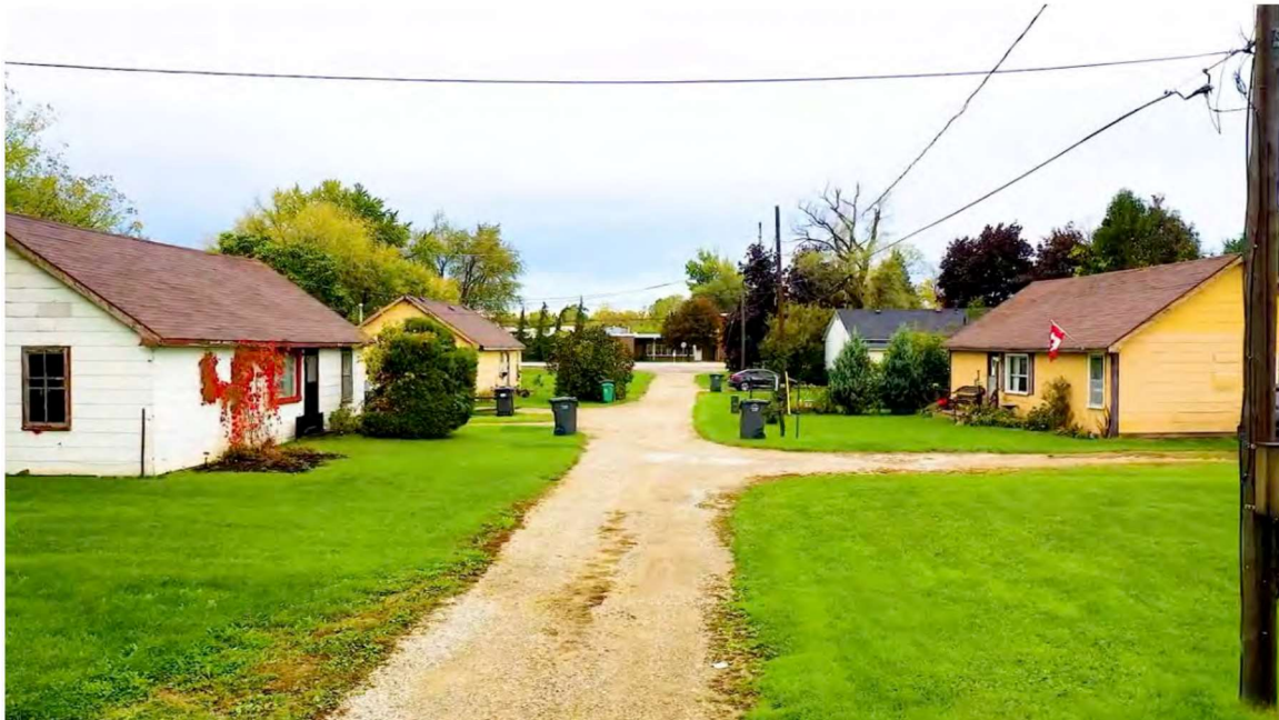
2305 Embleton Road – the subject property contains five one-storey dwellings on a private road dating from the second half of the 20 th century
