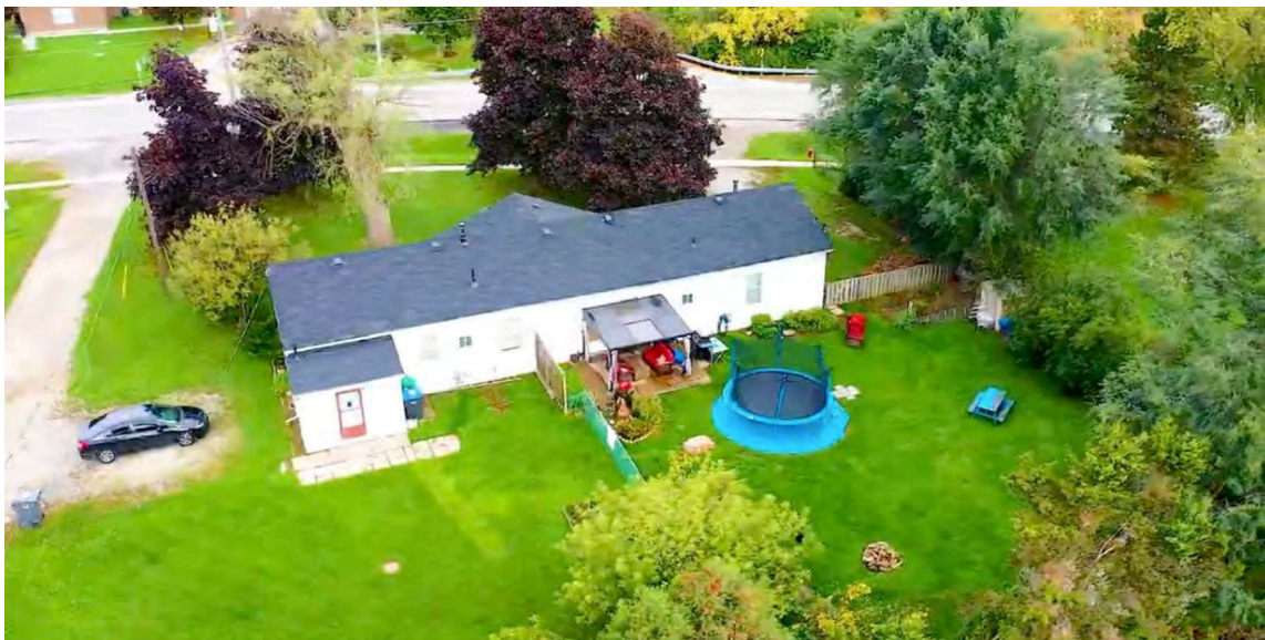
2305 Embleton Road – rear elevation of 20 th century dwelling on the subject property that faces Embleton Road
