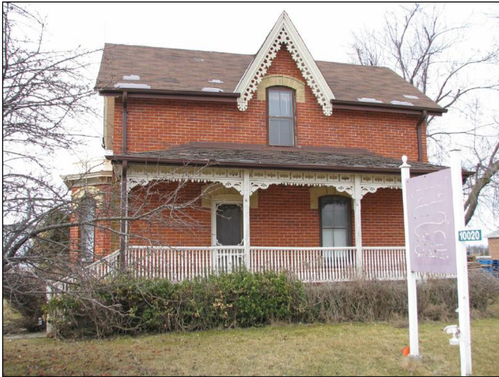
The building is a vernacular styled residence with Gothic Revival detailing with a centre gable with decorative vergeboard and dichromatic detailing over the window and door openings.
