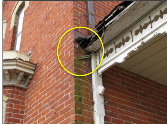
The circle indicates the location of markings brickwork on the south end of the verandah indicating an earlier verandah.
