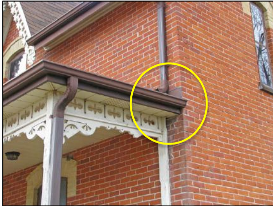
The circle indicates the location of markings brickwork on the north end of the verandah indicating an earlier verandah.
