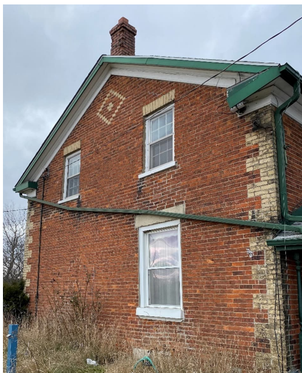
Plate 12: Example of flat arch window openings on the south elevation (Detail 1.4 in Figure 6)
