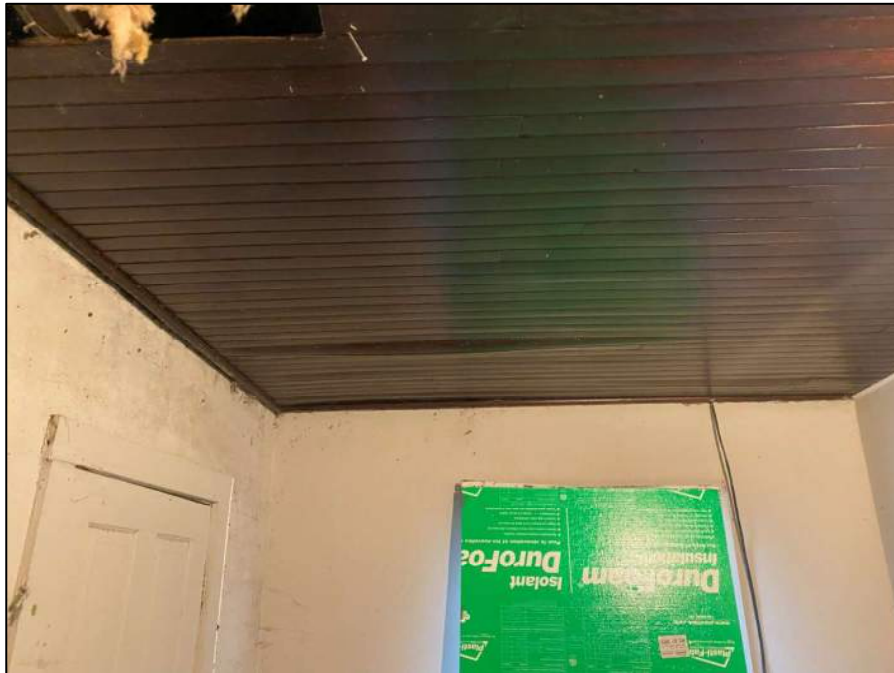
Photograph 5: Water damage to ceiling finishes
