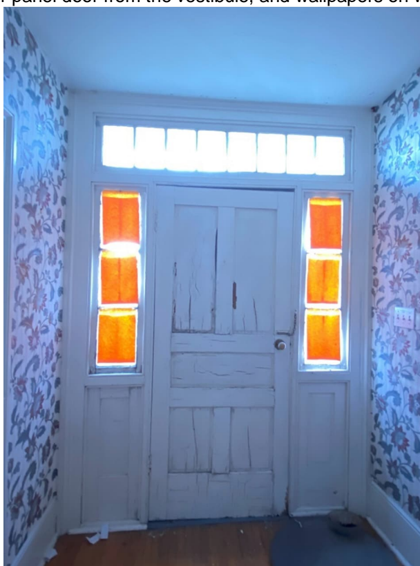
Plate 19: Single-leaf four panel door from the vestibule, and hardwood strip flooring (View B in Figure 8)
