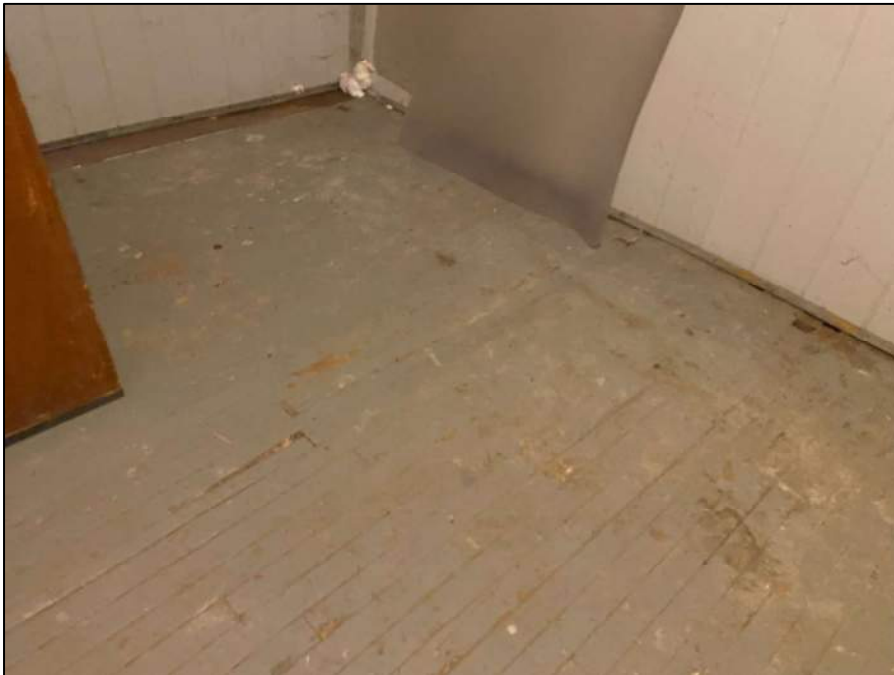
Photograph 6: Water damage to floor finishes
