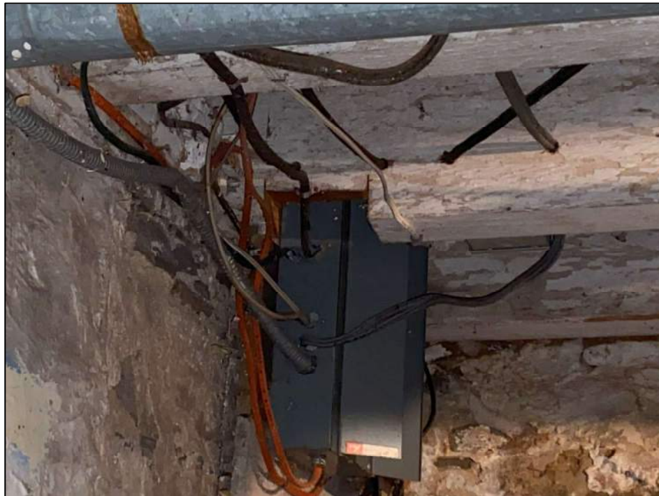
Photograph 3: Notched joist behind furnace
