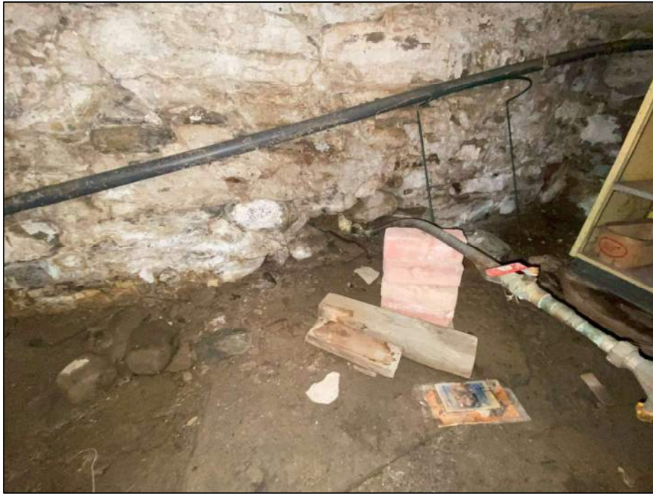
Photograph 4: Undermined section of foundation wall
