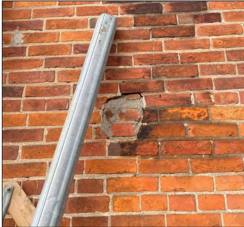
Photograph 10: Repair of past holes
