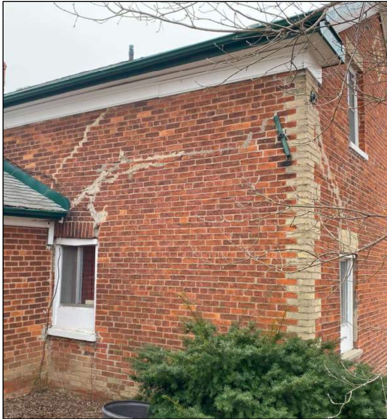
Photograph 8: Typical condition of exterior walls
