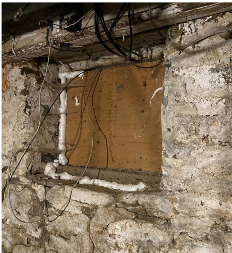
Plate 42: Coursed fieldstone foundation, facing west (View Y in Figure 10)
