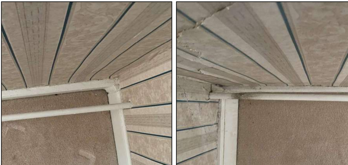
Photograph 1a & b: Relative deflection of wall based on offset from tension rod
