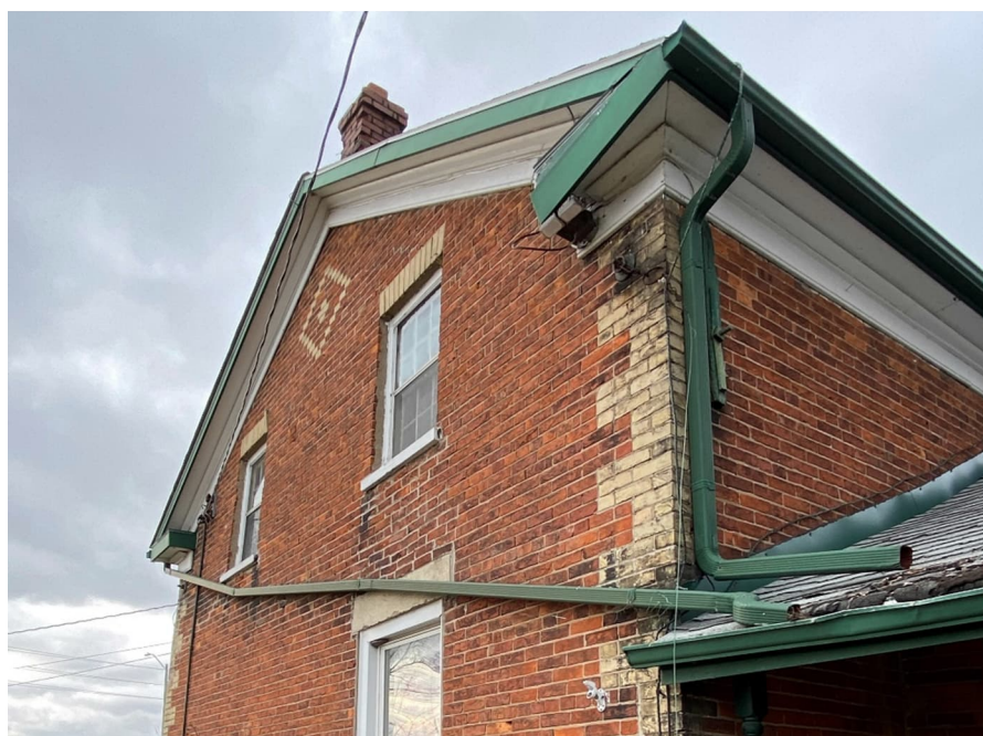
Plate 14: Medium gable roof, projecting eaves, verges with moulded soffit, plain fascia (Detail 1.5 in Figure 6)
