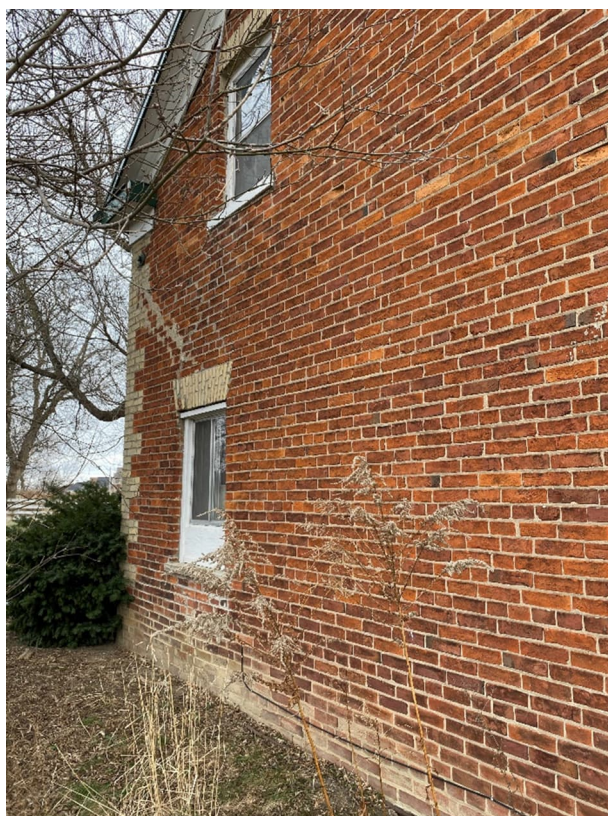
Plate 8: Window at first level, flat arch with plain trim, wide buff brick voussoirs, and stone lug sills, second-level, plain trim, flat arch buff brick headers, and plain lug sills (Detail 1.2 in Figure 5)
