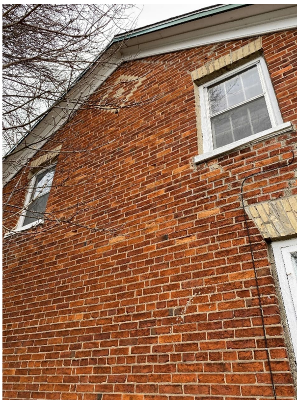
Plate 9: Buff brick decorative diamonds located below the gable (Detail 1.3 in Figure 5)
