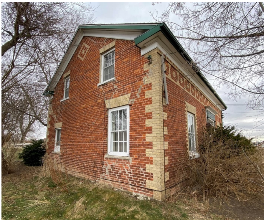
Plate 16: Buff brick quoins on north and west elevations (Detail 1.6 in Figure 4)
