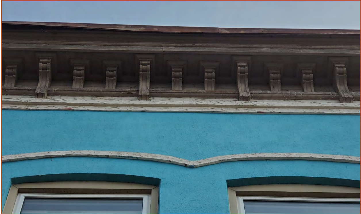
Photo 10. View northeast showing the corbel and frieze
