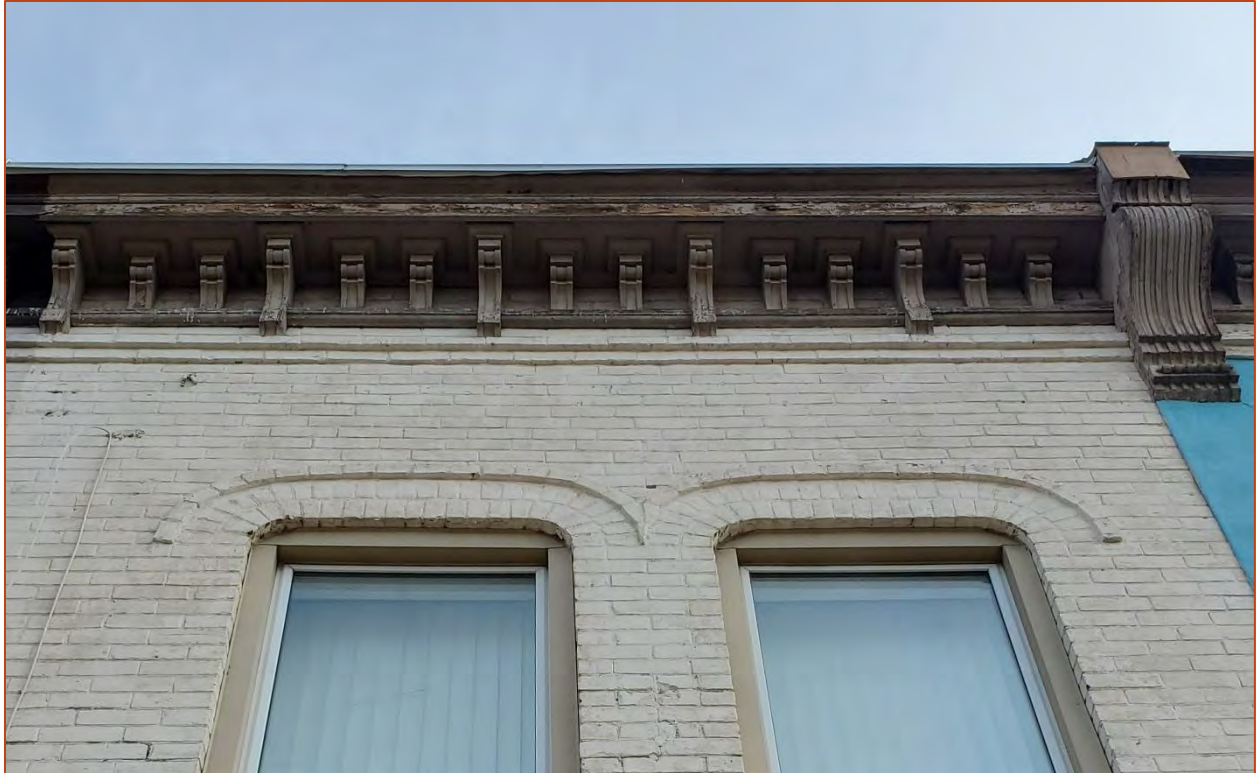
Photo 24. View northeast showing the corbel and frieze
