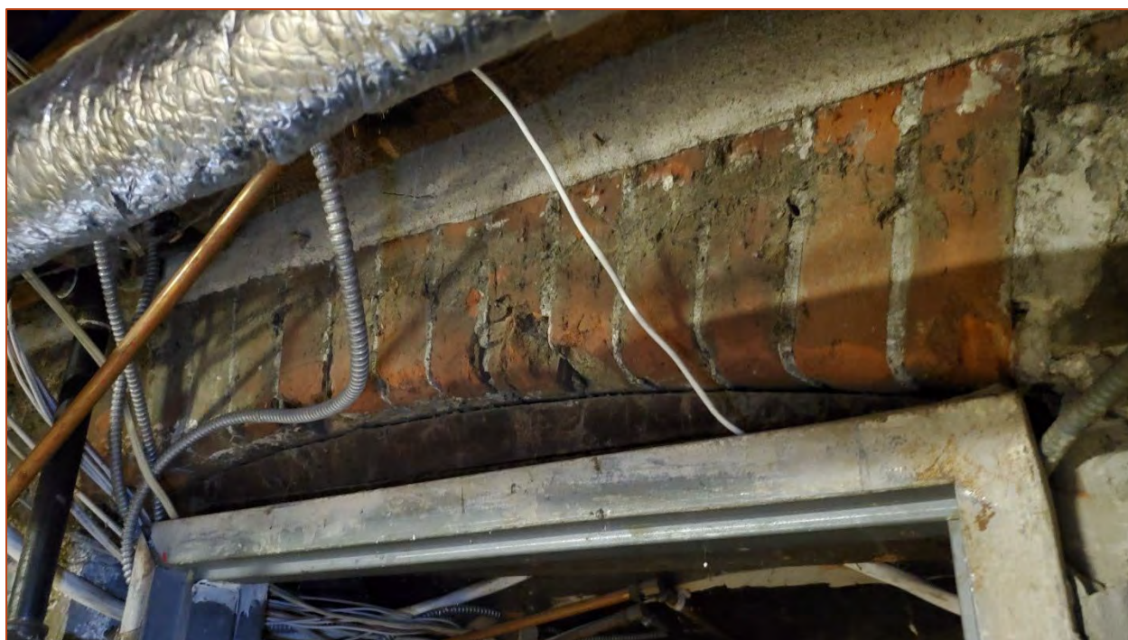
Photo 45. View southwest showing the voussoir over the door provided access between the centre and northeast rooms in the basement
