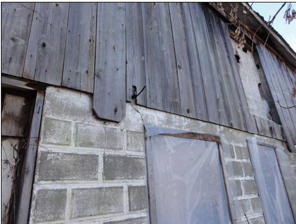
Plate 56: Concrete block foundations on east elevation.
