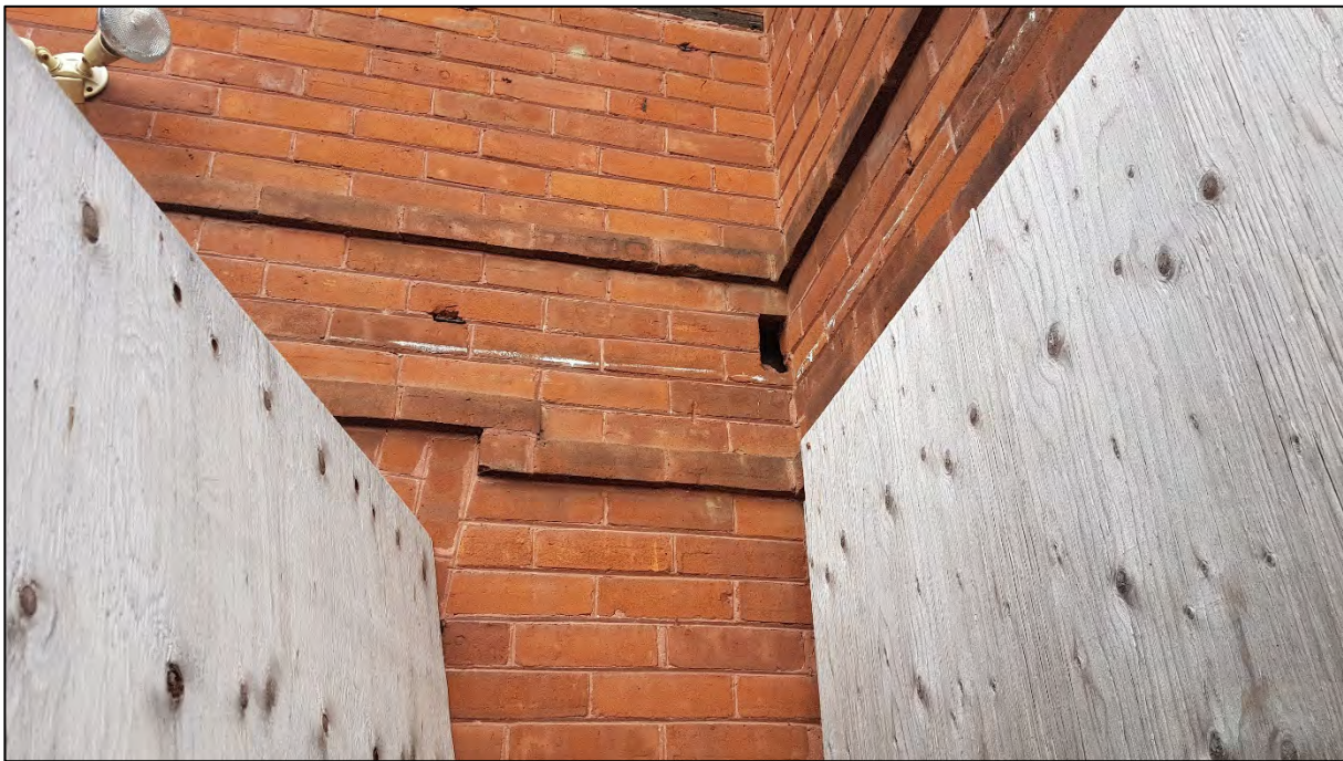
Figure 22: Joist hole where the original porch roof connected to the farmhouse (ASI 2020)
