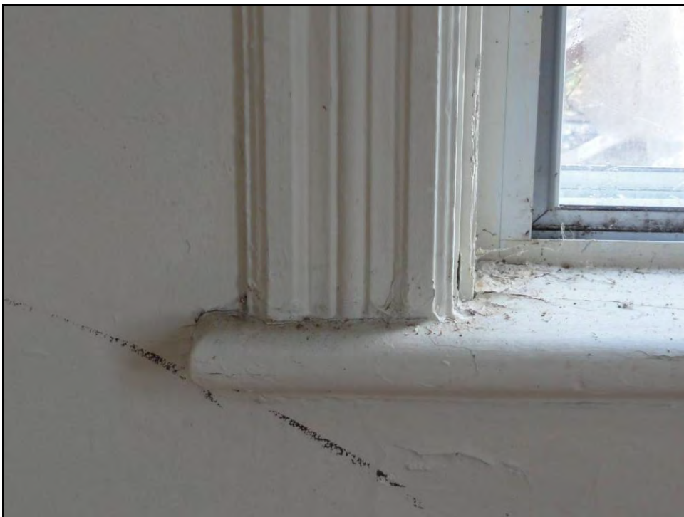
Plate 46: Fluted window casing with simple sill and no sill apron.
