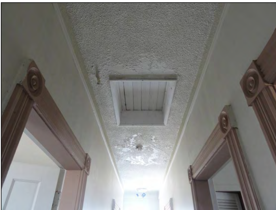
Plate 32: Access to the attic. Note the decorative casing around the doorways to Bedrooms No. 1 and 2, and the Bathroom.
