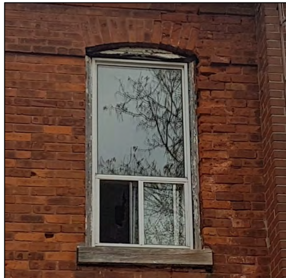
Figure 24: Second storey window showing the modern window with brick arch and wooden sill (ASI 2020)
