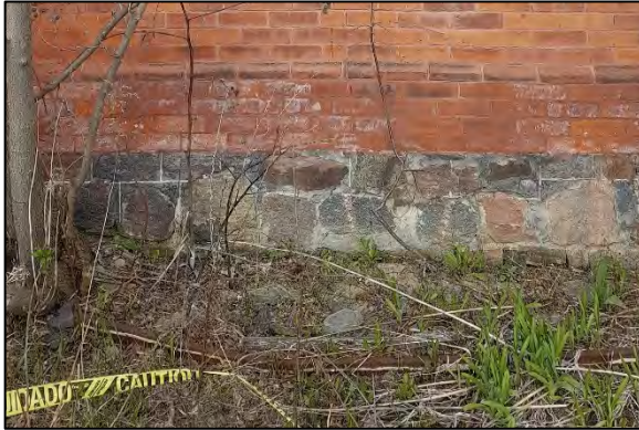
Figure 18: Granite foundations (ASI 2020)
