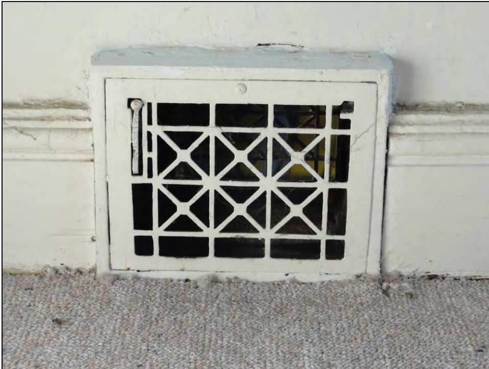
Plate 49: Note the heating grill in base of the wall and high, molded baseboards, located in Bedroom No.3.
