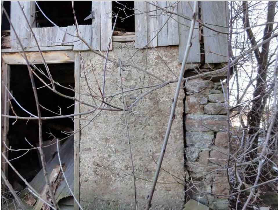
Plate 57: East elevation of barn, north corner, showing stone and poured concrete foundations.
