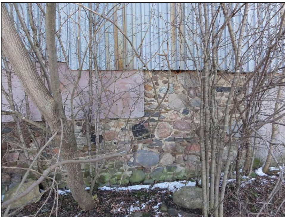
Plate 58: Detail of stone foundations on the north elevation, and blocked up windows.
