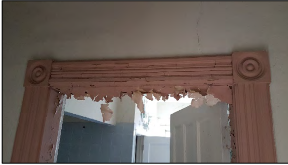
Figure 54: Mouldings around the door frames of the second-floor bedrooms (ASI 2020)
