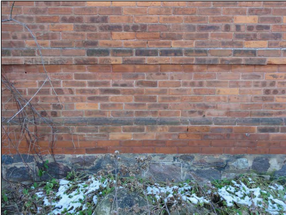
Plate 7: Detail of stone foundations, bands of projecting brick, and brick drip course above the foundations.
