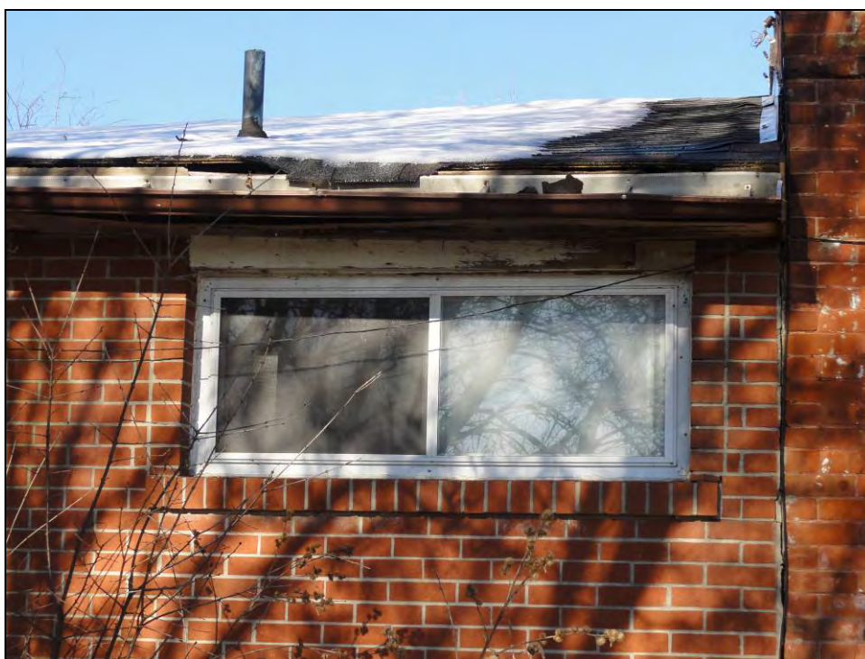
Plate 16: View of modern, side-sliding sash window in c.1960s rear accretion. Note the change in brickwork between front and back sections of the house.
