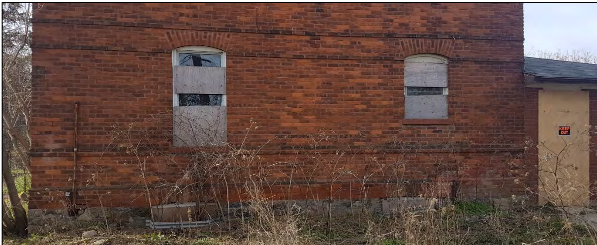
Figure 20: Brick bands on the north elevation (ASI 2020)
