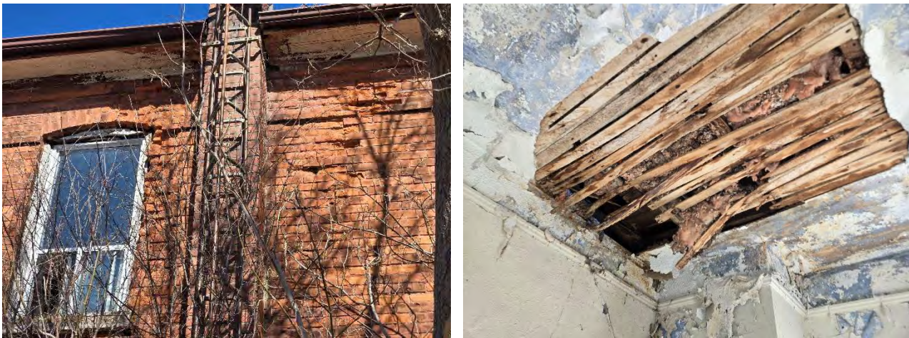
Photos 17-18- (above, left) View of south elevation noting condition of brick, (below, right) View of interior framing (second storey) noting condition of wood as a result of water egress (MHBC, 2025).
