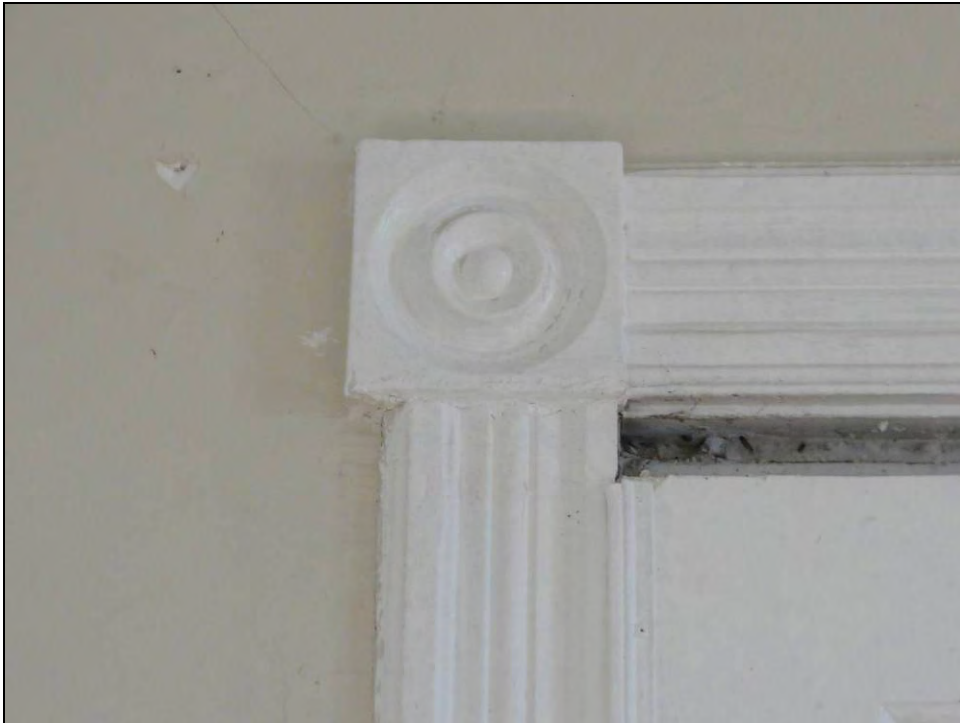
Plate 47: Bullseye rosette block at corner of front door casing in the den.
