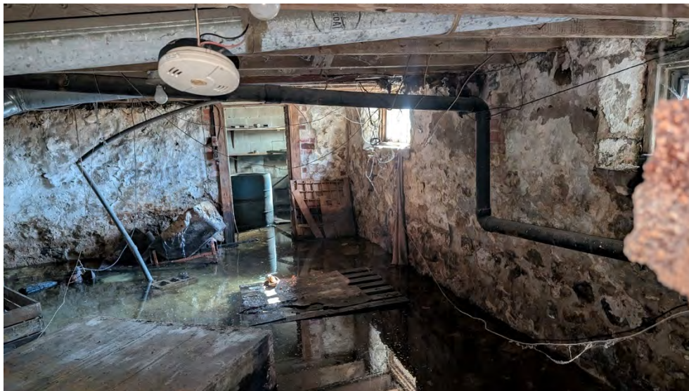
Photograph 3 – Flooded Basement
