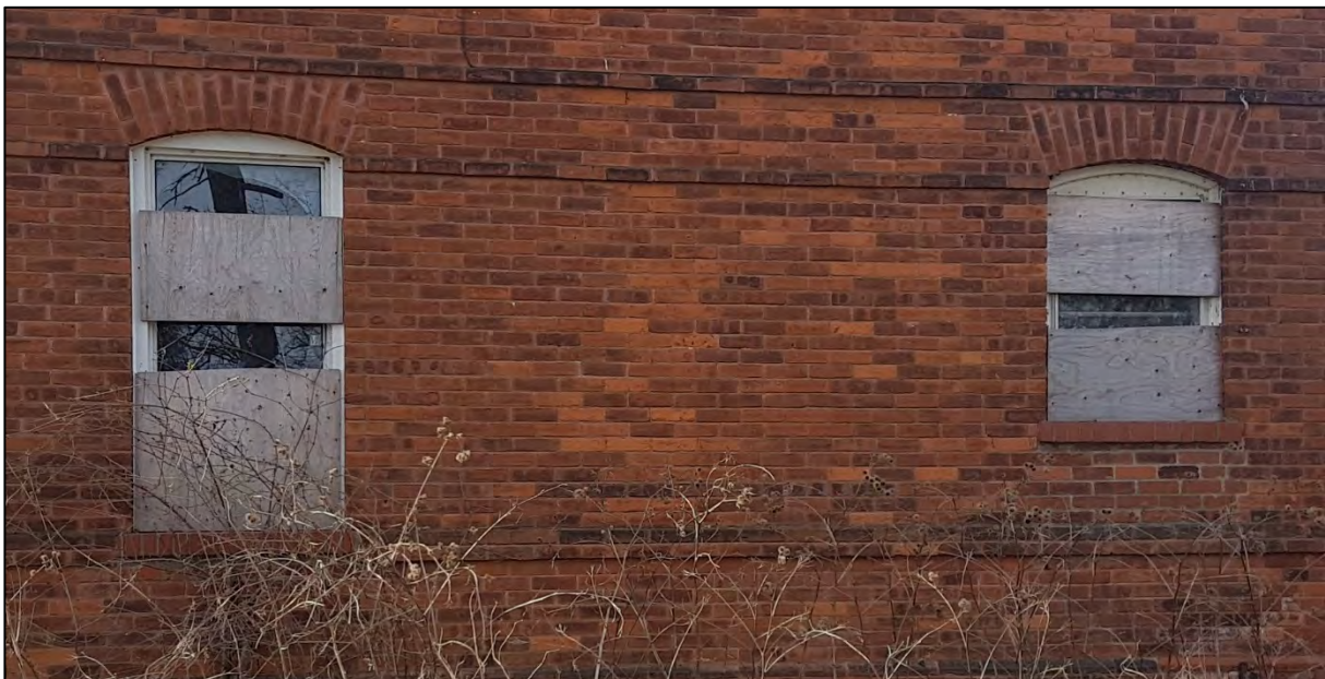
Figure 26: First storey windows with brick sills (ASI 2020)
