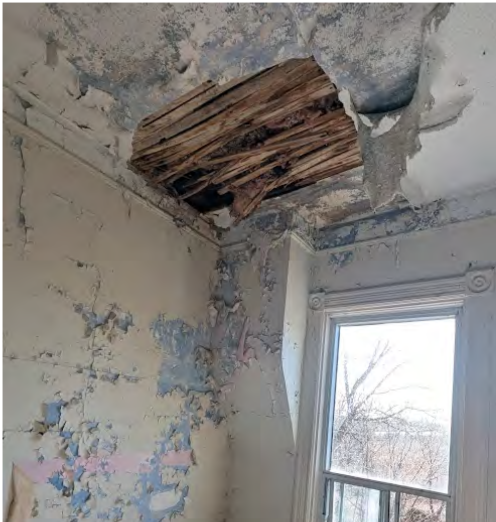
Photograph 2 - Interior Ceiling / Roof Collapse
