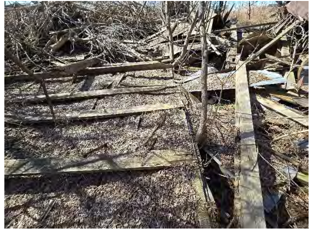
Photos 19-20- (above, left) View of collapse of interior structural beams of the barn, (below, right) View of collapsed barn framing materials, (MHBC, 2025).
