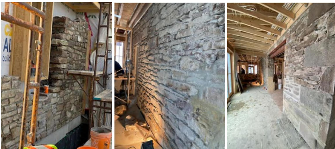
Figure 19: Process to create the masonry veneer. Left: framing complete before laying up veneer. Centre: Veneer laid up in mortar. Right: Grout applied for a uniform finish (subsequently acid treated) (from Robert Wilson House, Town of Caledon, courtesy Sedgwick Marshall Heritage Homes Ltd)
