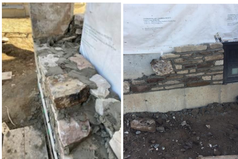
Figure 18: Ledge incorporated into the concrete foundation that provides a base for the exterior masonry wythe (from Robert Wilson House, Town of Caledon, courtesy Sedgwick Marshall Heritage Homes Ltd)
