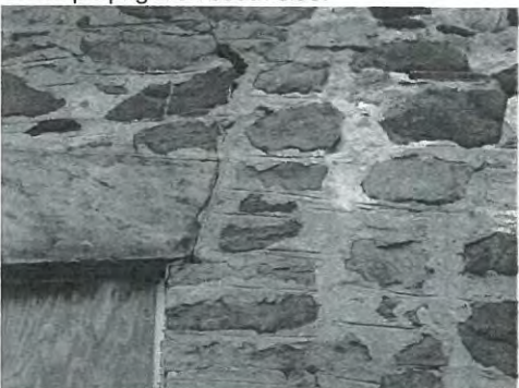
Crack propagation south side.
