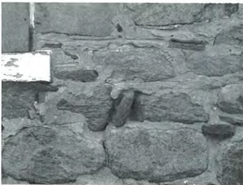
Mortar erosion, west side.
