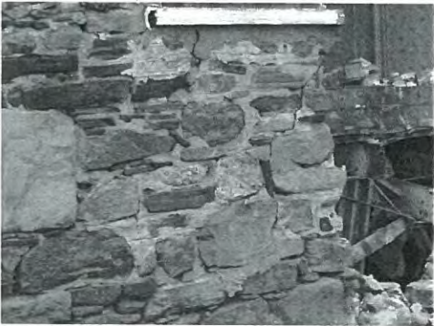
Crack propagation south side.
