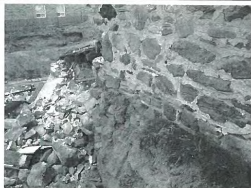
North side foundation, where salt-box joined. Even the intact foundation appears to be unconsolidated rubble.
