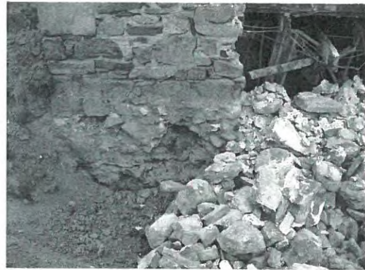
South side. Even material not involved in general failure has fallen away.
