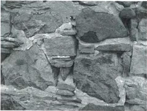
Mortar erosion, west side.
