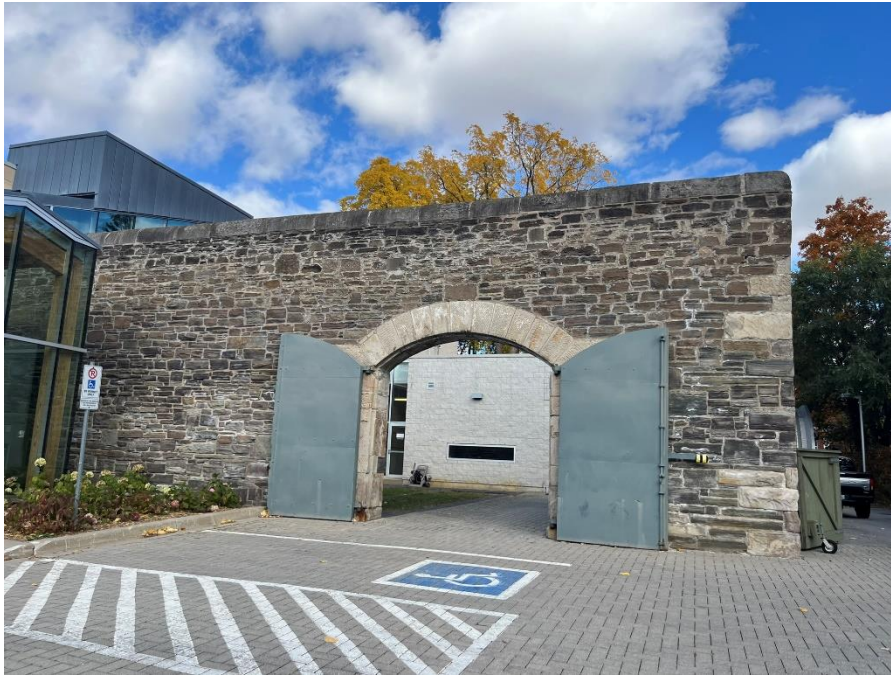
Figure 10: The yard wall at the Peel County Jail, constructed from stone from the former Kennedy Valley Quarry (A.S.I., 2024).
