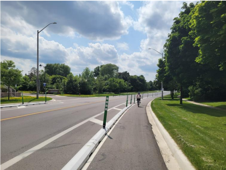
Protected on-road bike lane
