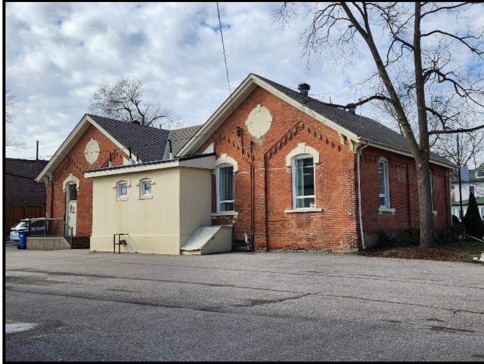
Image 5: East (Rear) Elevation of 147 Queen Street West (Photo taken February 7, 2024; Facing Southwest)
