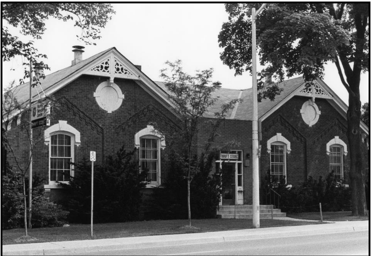
Figure 5: Façade of 147 Queen Street West When Operating as a Salvation Army Thrift Store (Circa 1970s or 1980s) (CoB 2014)
