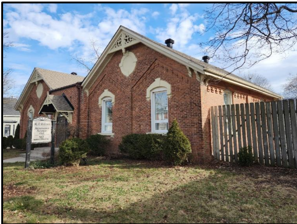
Image 6: Southwest Corner of 147 Queen Street West (Photo taken February 7, 2024; Facing Northeast)
