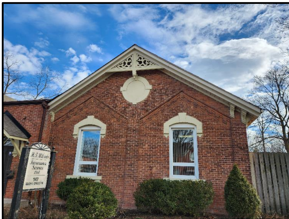
Image 2: Detail of Façade Bay and Gable of 147 Queen Street West (Photo taken February 7, 2024; Facing Southeast)
