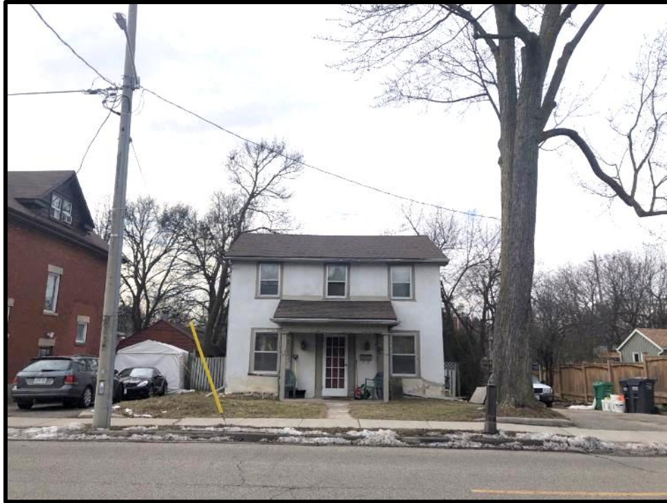
Image 5: Context View of 15 Isabella Street (Photo taken February 7, 2024; Facing Southwest)
