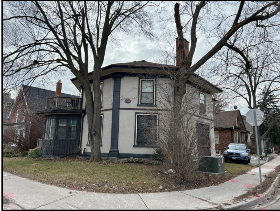
Image 1: Façade of 227 Main Street North (Photo taken February 7, 2024; Facing South)
