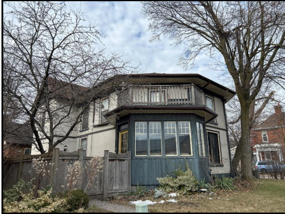
Image 3: Northeast Corner of 227 Main Street North (Photo taken February 7, 2024; Facing West)
