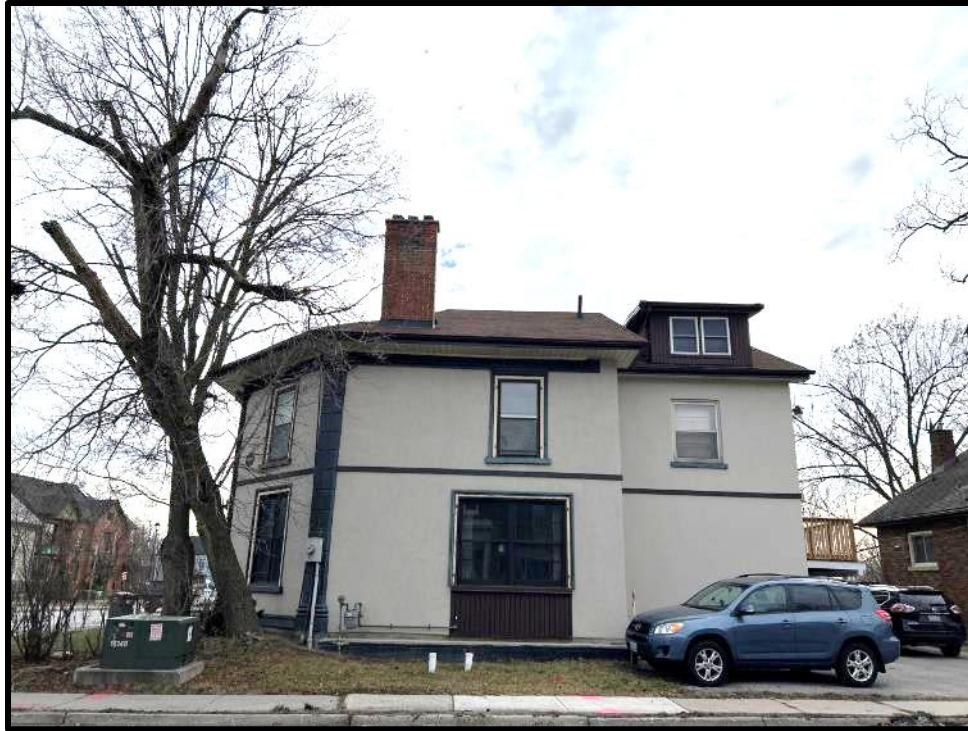
Image 7: West Elevation of 227 Main Street North (Photo taken February 7, 2024; Facing Southeast)
