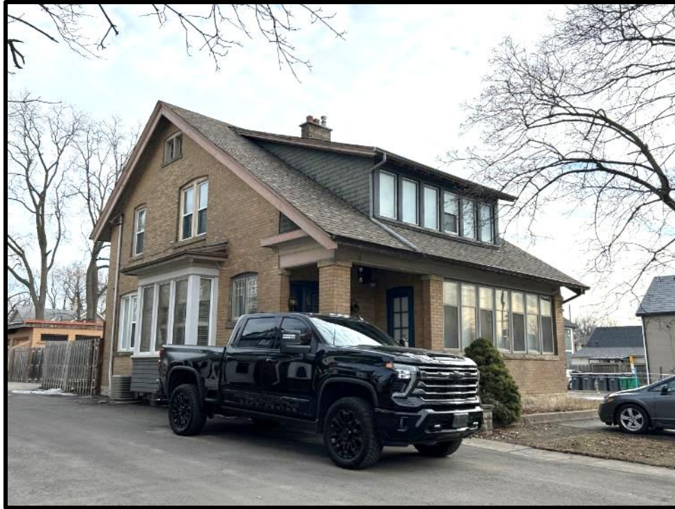
Image 3: Southwest Corner of 230 Main Street North (Photo taken February 7, 2024; Facing East)
