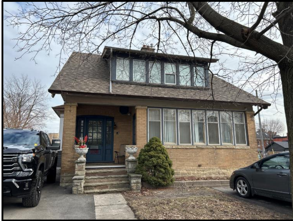
Image 1: South Façade of 230 Main Street North (Photo taken February 7, 2024; Facing Northeast)
