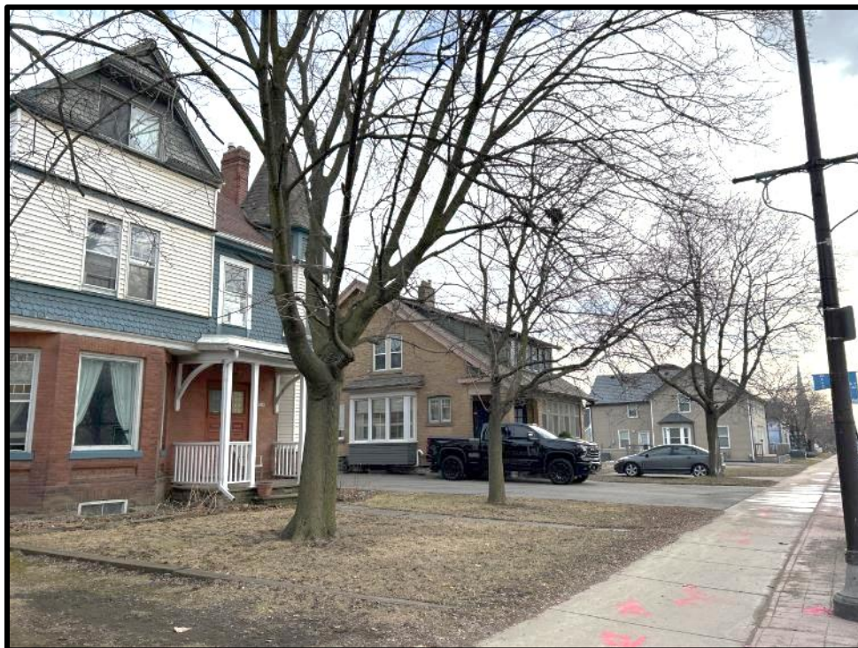
Image 6: Context View of Main Street North Looking Toward 230 Main Street North (Photo taken February 7, 2024; Facing Southeast)
