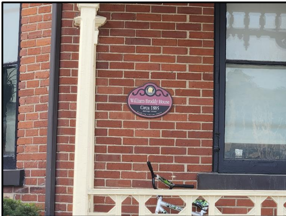
Image 6: Detail of Plaque on Façade of 243-245 Main Street North (Photo taken February 7, 2024; Facing Southwest)
