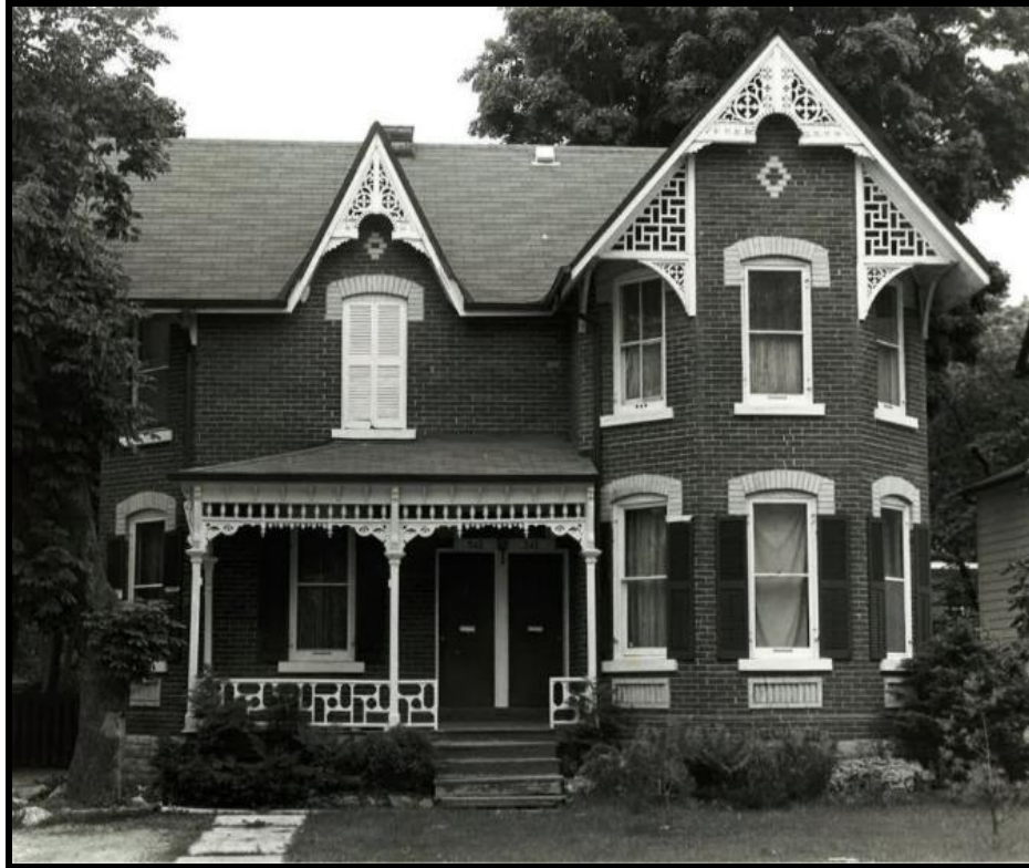
Figure 5: Façade of 243-245 Main Street North (n.d.) (CoB n.d.)
