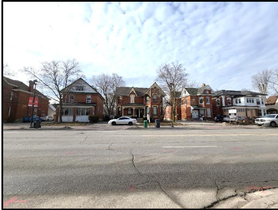
Image 9: Context View of 243-245 Main Street North From Main Street North (Photo taken February 7, 2024; Facing Southwest)
