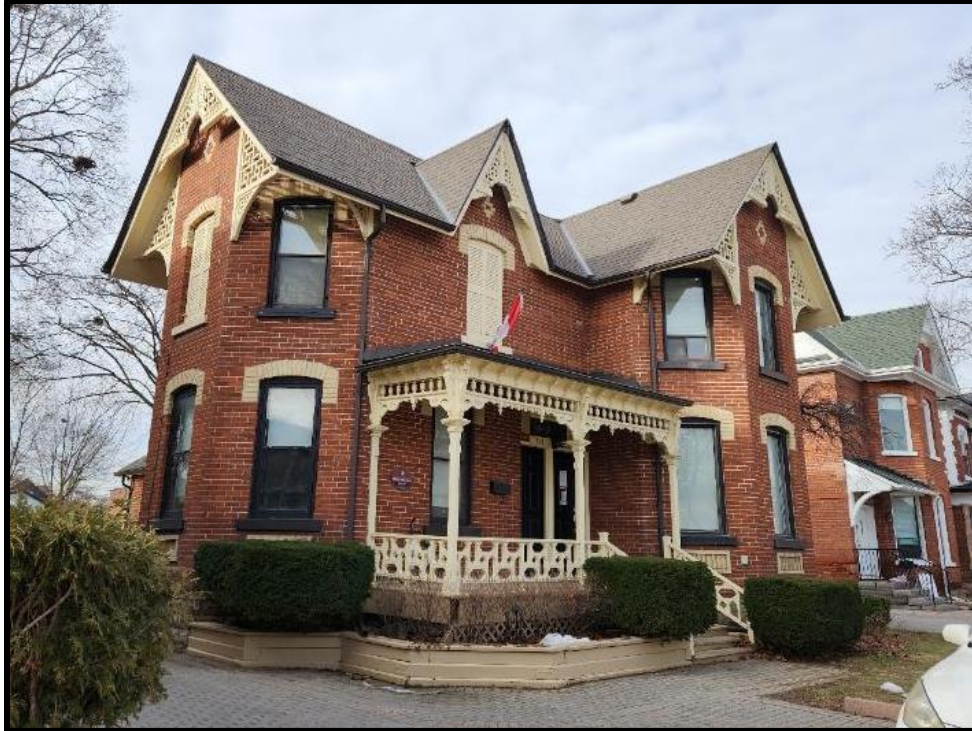
Image 7: Northeast Corner of 243-245 Main Street North (Photo taken February 7, 2024; Facing West)
