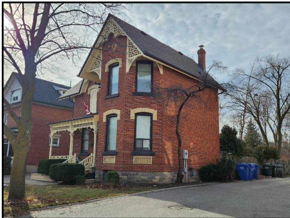
Image 8: Northwest Corner of 243-245 Main Street North (Photo taken February 7, 2024; Facing Southeast)
