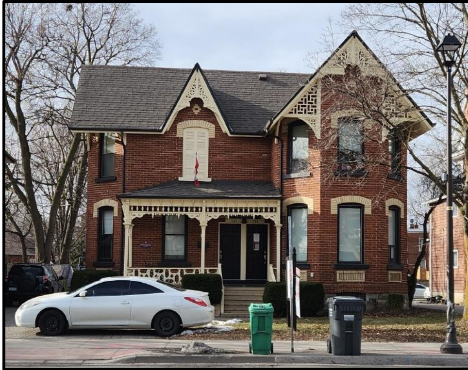
Image 1: North Façade of 243-245 Main Street North (Photo taken February 7, 2024; Facing Southwest)
