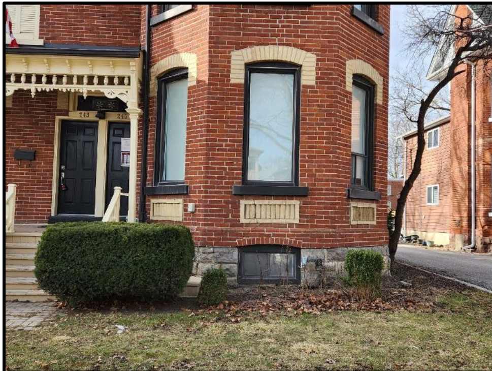
Image 4: Projecting Bay of 243-245 Main Street North (Photo taken February 7, 2024; Facing Southwest)
