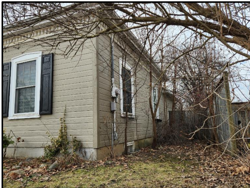
Image 6: Northwest Corner of 3 Isabella Street (Photo taken February 7, 2024; Facing South)
