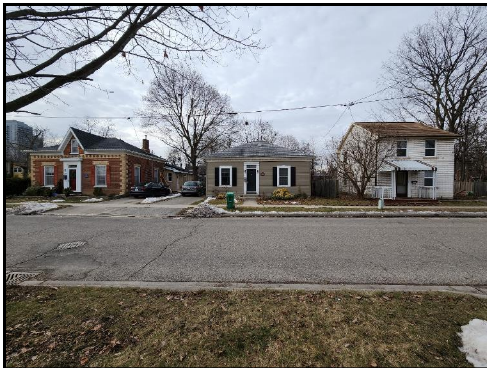
Image 8: Context View of 3 Isabella Street from North Side of Isabella Street (Photo taken February 7, 2024; Facing Southwest)
