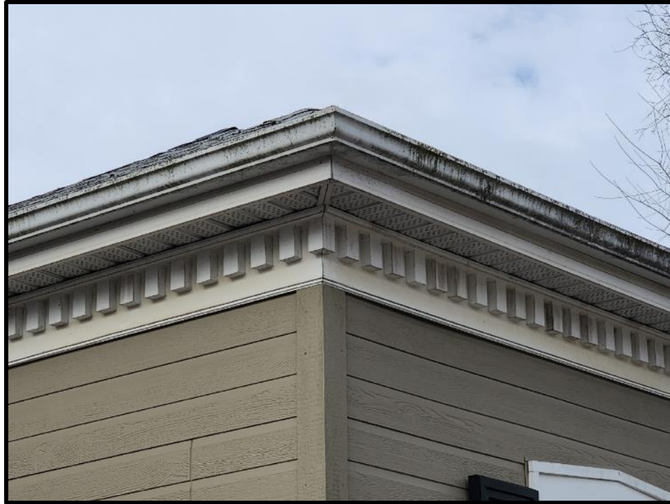
Image 5: Detail of Cornice of 3 Isabella Street (Photo taken February 7, 2024; Facing West)
