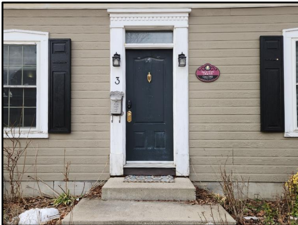
Image 2: Detail of Entryway of 3 Isabella Street (Photo taken February 7, 2024; Facing Southwest)
