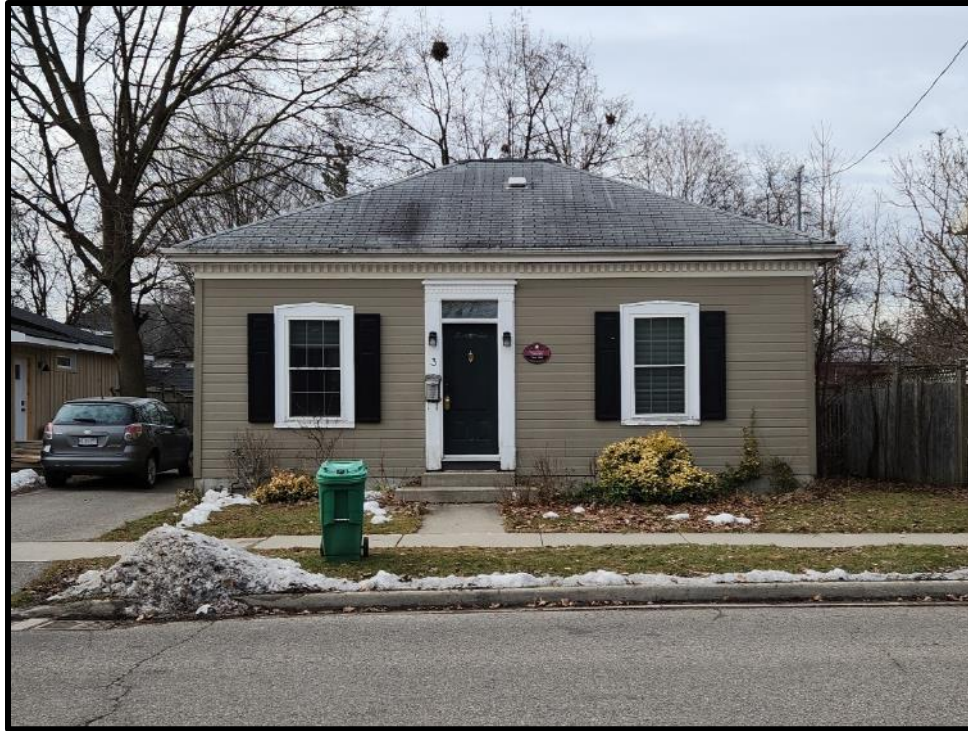
Image 1: Façade of 3 Isabella Street (Photo taken February 7, 2024; Facing Southwest)
