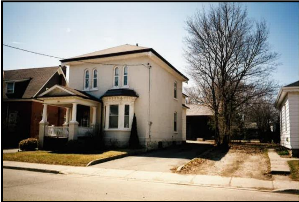
Figure 1: Image of 35 Elizabeth Street North (Date Unknown) (CoB n.d.a)
