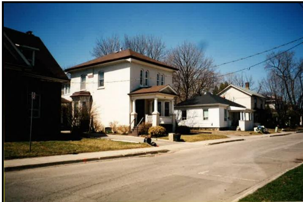
Figure 3: Image of 35 Elizabeth Street North (Date Unknown) (CoB n.d.a)
