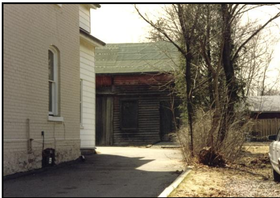
Figure 4: Image of Driveshed in Rear of Property at 35 Elizabeth Street North (Date Unknown) (CoB n.d.a)
