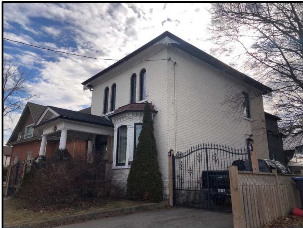
Image 6: West Elevation of 35 Elizabeth Street North (Photo taken February 7, 2024; Facing South)
