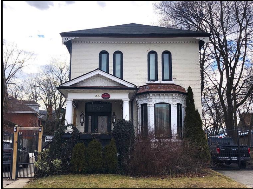
Image 1: Façade of 35 Elizabeth Street North (Photo taken February 7, 2024; Facing Southwest)
