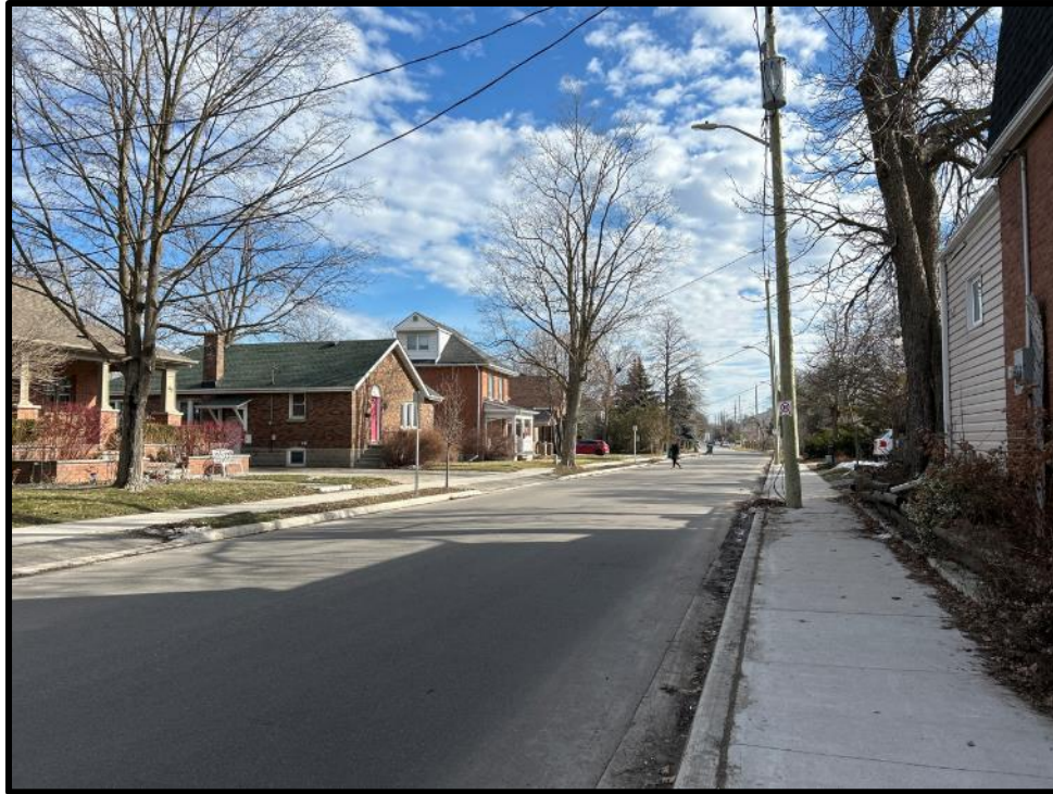
Image 9: Context View of Elliott Street From Fleming Avenue (Photo taken February 7, 2024; Facing Southeast)
