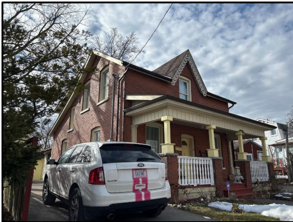
Image 4: Northeast Corner of 41 Elliott Street (Photo taken February 7, 2024; Facing West)
