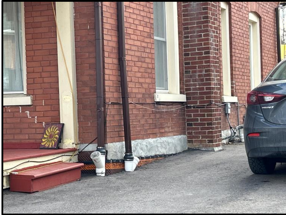
Image 7: Detail of Foundation of 41 Elliott Street (Photo taken February 7, 2024; Facing South)
