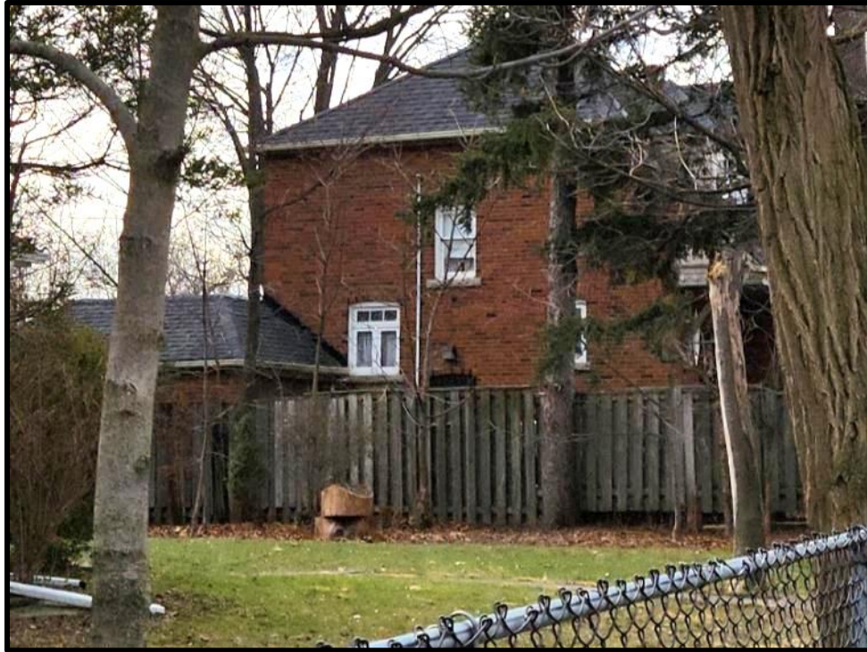
Image 5: North Elevation of 51 David Street (Photo taken February 7, 2024; Facing South)
