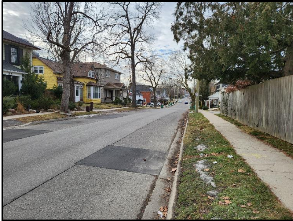
Image 9: Context View of David Street From Near Isabella Street (Photo taken February 7, 2024; Facing Southwest)
