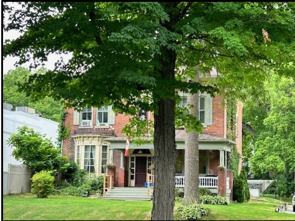
Image 5: Southeast Corner of 56 Main Street South (Photo taken August 8, 2024; Facing North)
