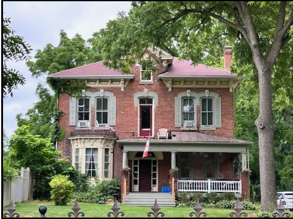
Image 1: Façade of 56 Main Street South (Photo taken August 8, 2024; Facing Northeast)
