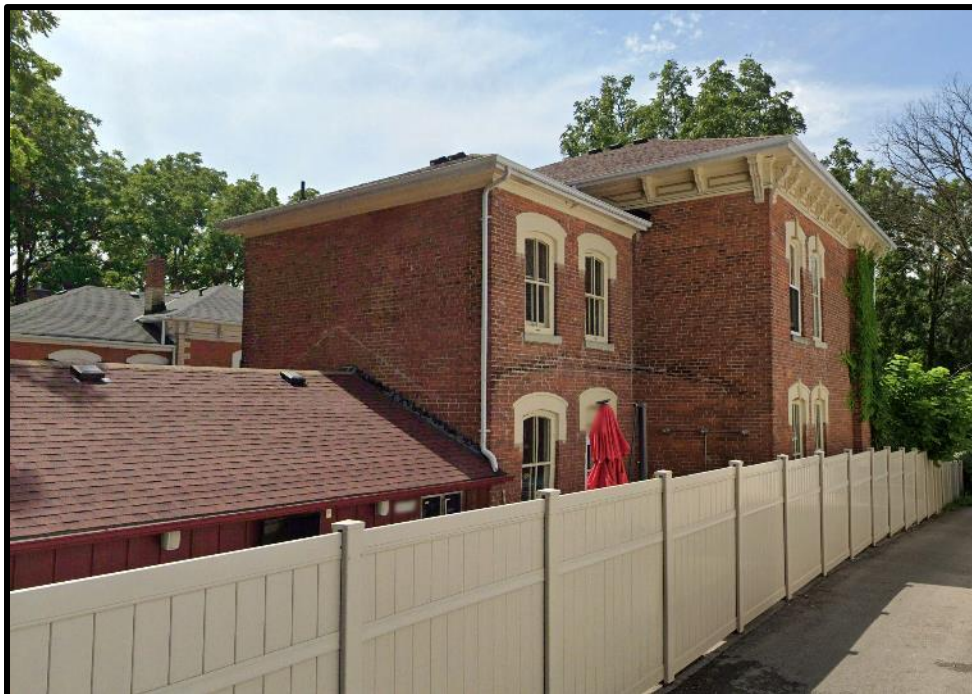
Image 4: Northwest Corner of 56 Main Street South (Google Earth 2022; Facing South)
