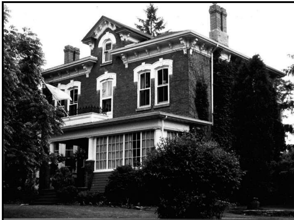
Figure 12: Southeast Corner of 56 Main Street South (Date Unknown) (CoB n.d.a)
