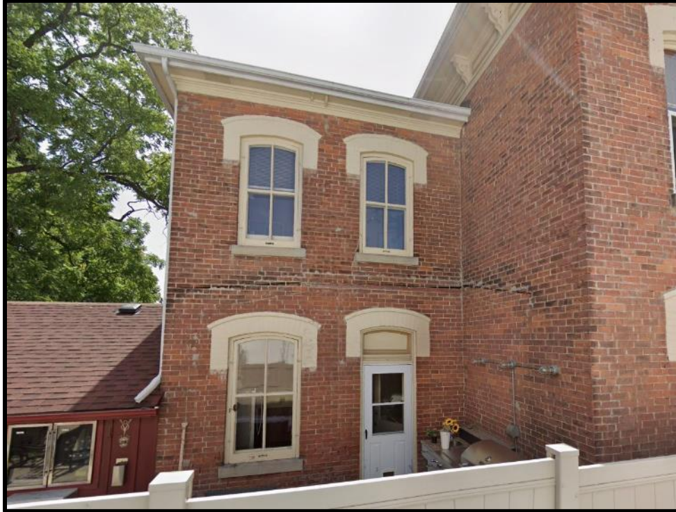
Image 3: West Elevation of Two-Storey Rear Wing of 56 Main Street South (Google Earth 2022; Facing East)
