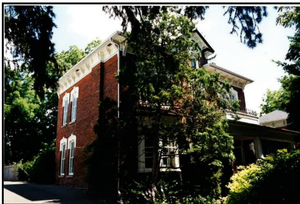
Figure 15: West Elevation of 56 Main Street South (Date Unknown) (CoB n.d.c)
