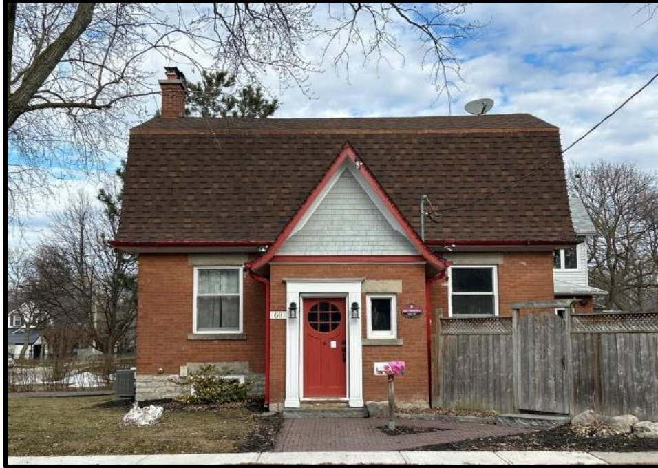
Image 1: South Façade of 60 Mill Street South (Photo taken February 7, 2024; Facing Northeast)
