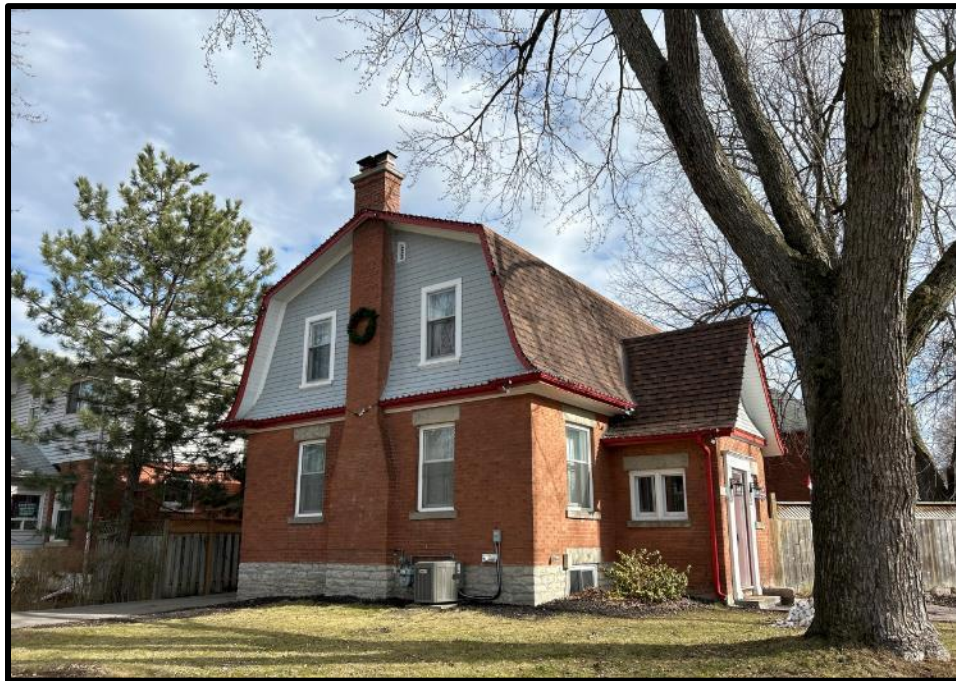
Image 2: Southwest Corner of 60 Mill Street South (Photo taken February 7, 2024; Facing East)
