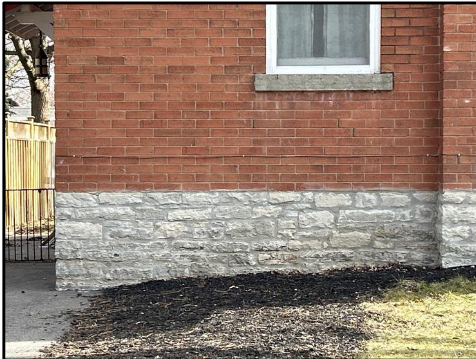
Image 6: Detail of Stone Foundation of 60 Mill Street South (Photo taken February 7, 2024; Facing East)
