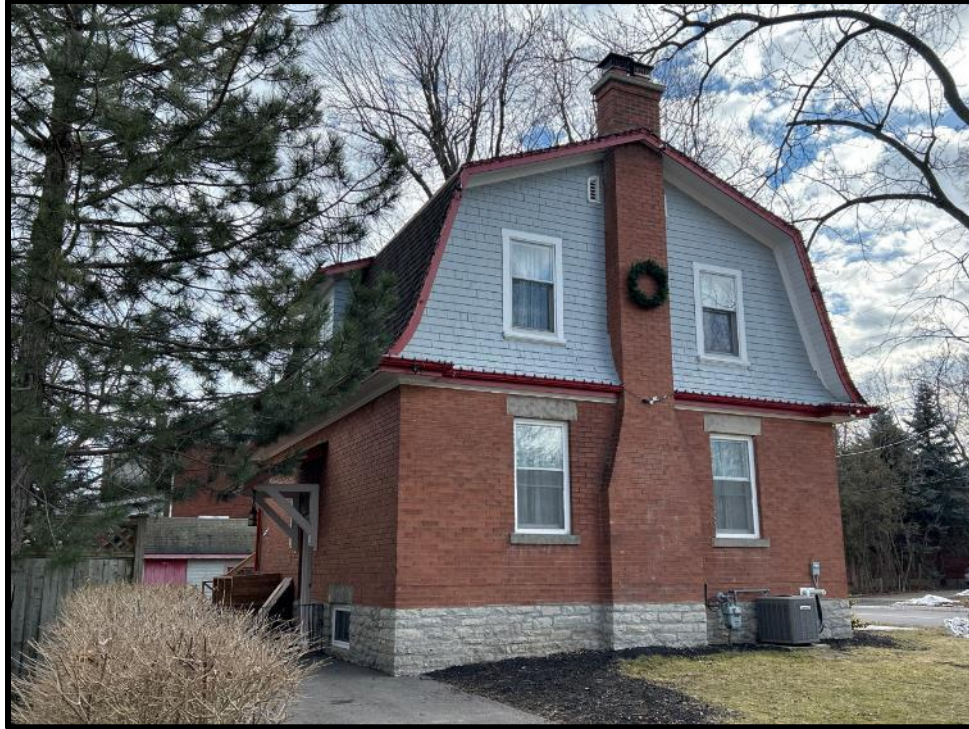
Image 5: Northwest Corner of 60 Mill Street South (Photo taken February 7, 2024; Facing Southeast)
