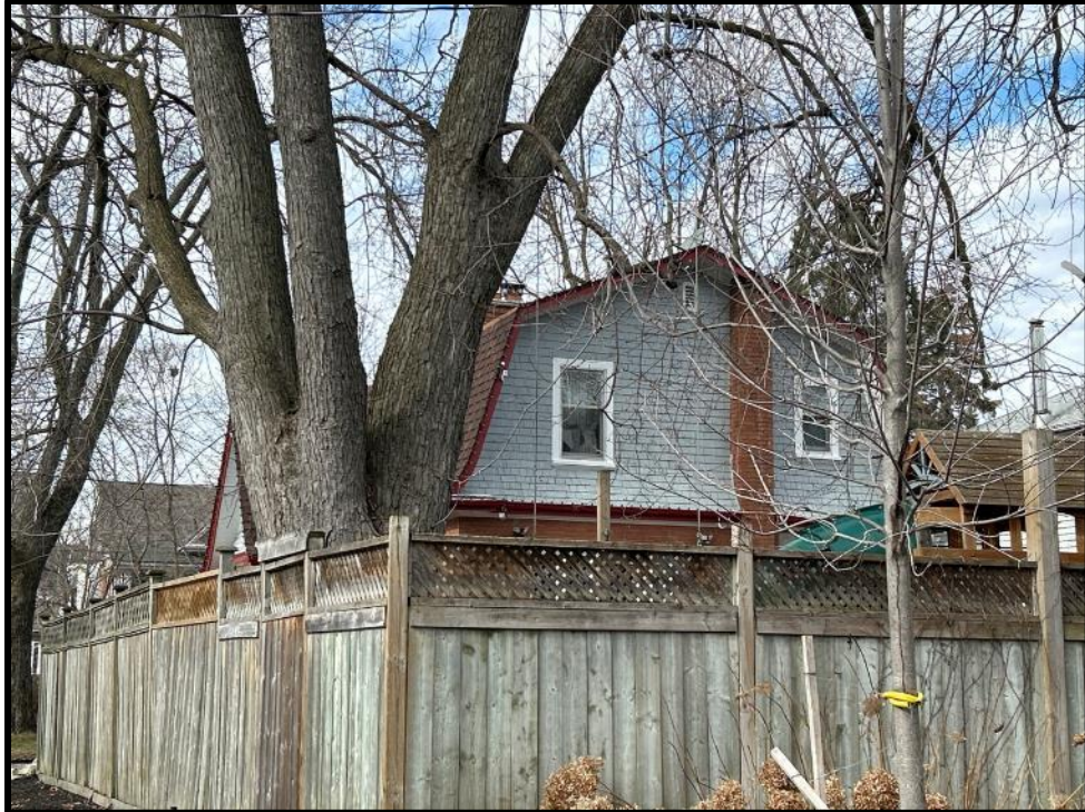
Image 7: East Elevation of 60 Mill Street South (Photo taken February 7, 2024; Facing Northwest)
