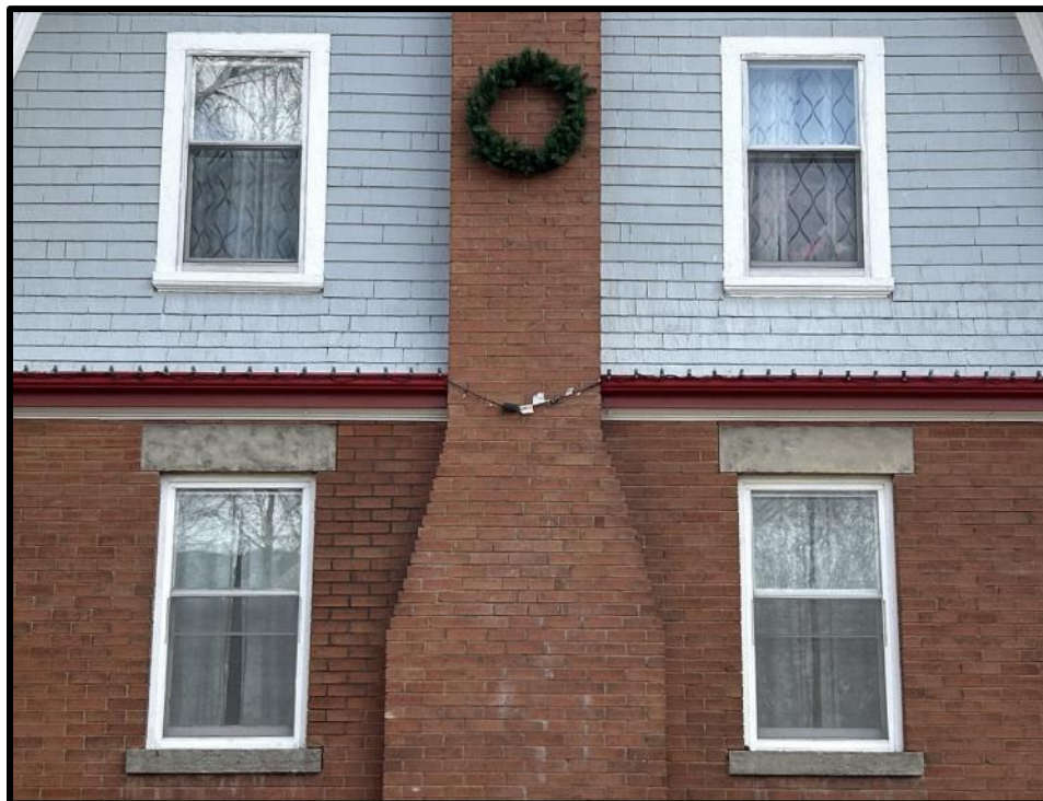
Image 4: Detail of West Elevation of 60 Mill Street South (Photo taken February 7, 2024; Facing East)
