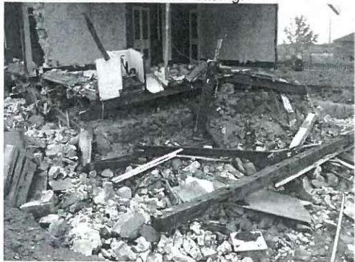
View of southeast corner of salt-box.
