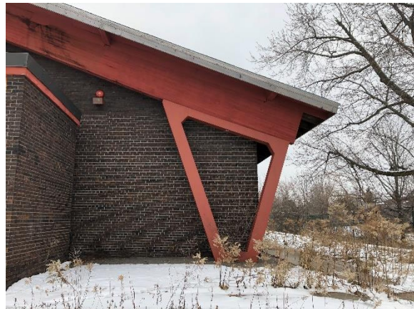
Image 8: View of the concrete pillar supporting the glulam beam, note all concrete pillars are of this shape, but the other concrete pillars are partially enclosed inside the building.
