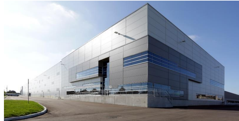
8875 Torbram Rd.(Complete 2015). Occupied by MEC, TJX, Accuristix. 994,000 sf, 38 ft Clear Heights.
