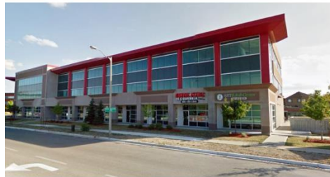
Sunny Meadows Condominium Office, 54,000 sf
