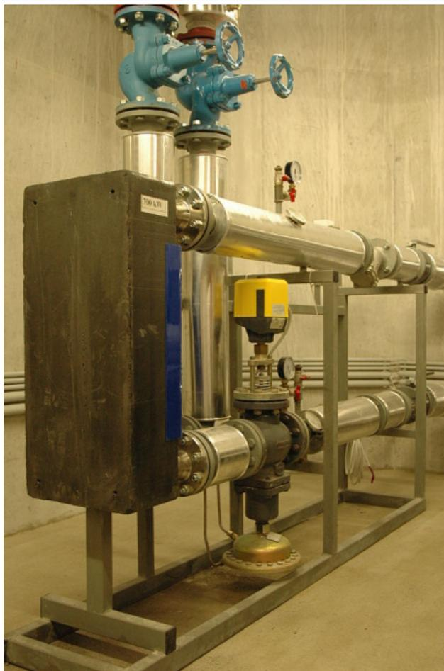
Figure D12.1- Example of District Heating Substation
