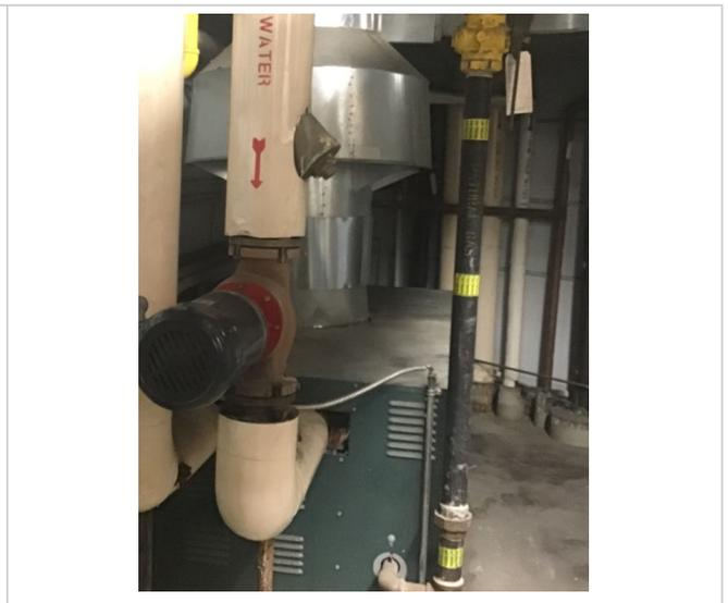
Figure D01.2 – Existing Atmospheric Boiler
