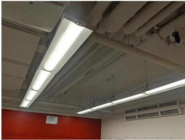
Figure A03.1 – Typical lighting layout in a change room. Occupancy sensor to be placed in center of room.
