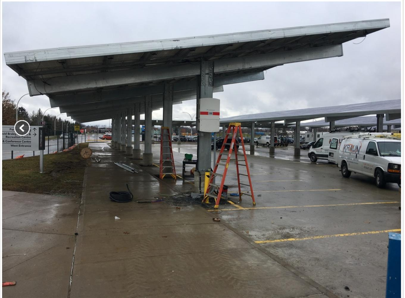
Figure I02.2: : Proposed solar carport support structure, similar array installed at Mohawk College, Hamilton
