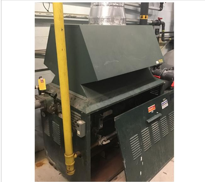
Figure D03.1 – Existing Atmospheric Pool Boiler
