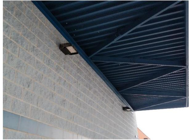
Figure A02.2 – LED wall pack replacements
