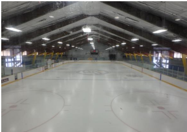
Image 28: View of the ice rink in February 2016, prior to the fire (City of Brampton, 2020).
