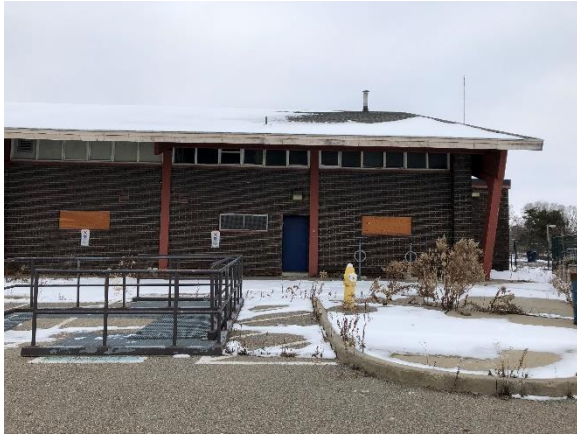
Image 15: View of the front section of the southeast side elevation.
