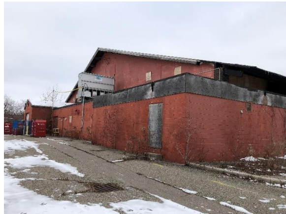
Image 18: View of the rear elevation from the southmost corner.
