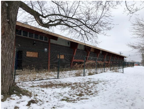
Image 11: View of the northwest side elevation.
