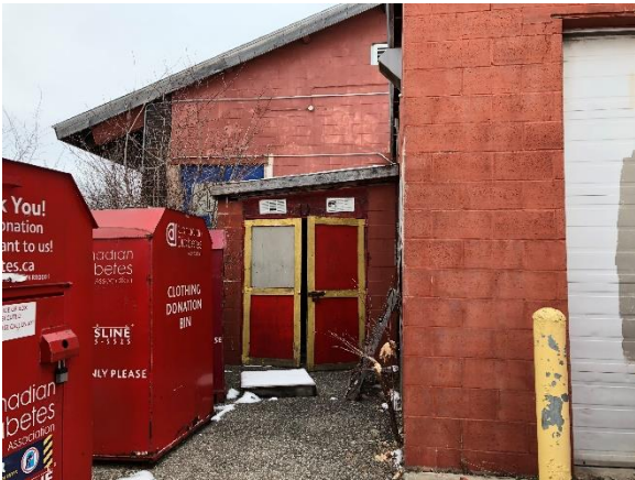
Image 24: View of a small shed attached to the rear elevation.
