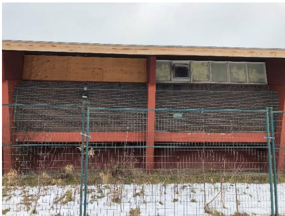
Image 13: View of a section of the northwest side elevation.
