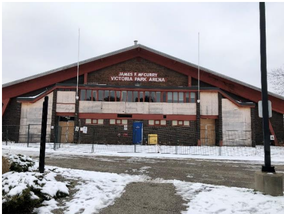
Image 7: View of the projecting portion on the front elevation of Victoria Park Arena.
