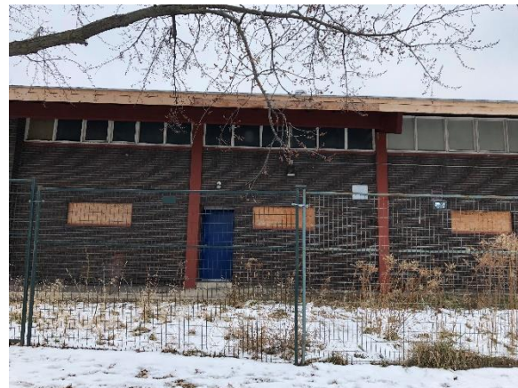
Image 14: View of the front section of the northwest side elevation.
