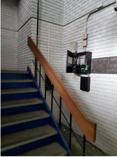
Image 30: View of the stairs at the front of the building leading to the viewing area on the second floor.
