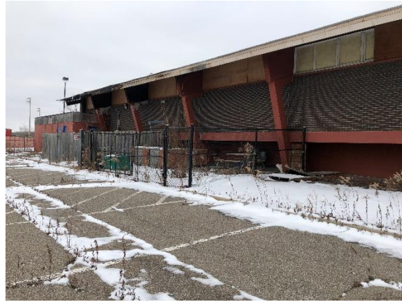
Image 16: View of the southeast side elevation towards the rear of the building.
