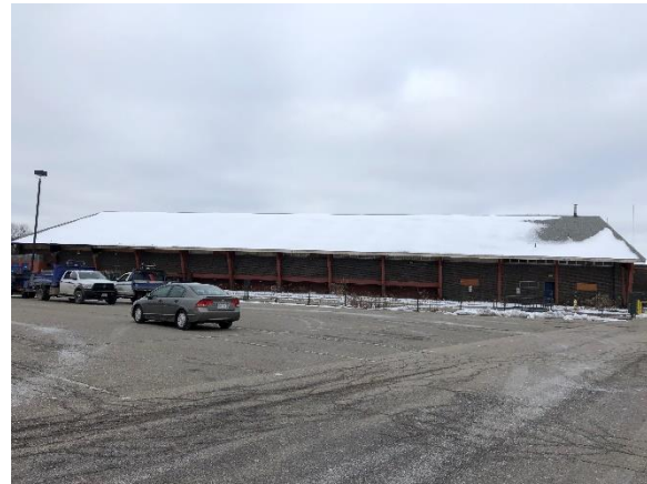
Image 12: View of the southeast side elevation.
