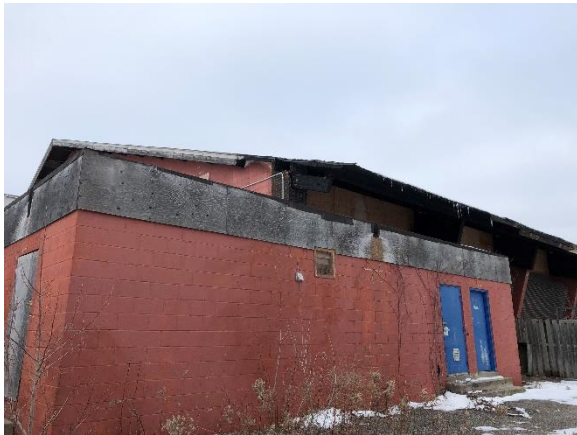
Image 19: View of the southeast side of one of the rear additions.
