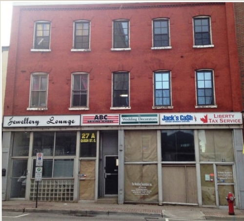
23-27 Queen Street East before façade improvement
