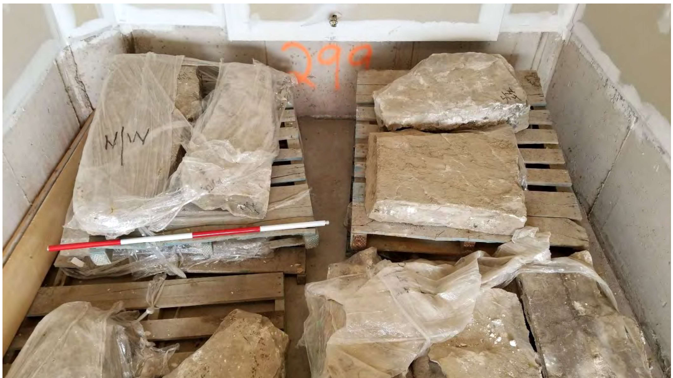
Figure 21: Stones from the north and west façade of Breadner House being stored off-site (November 2019)
