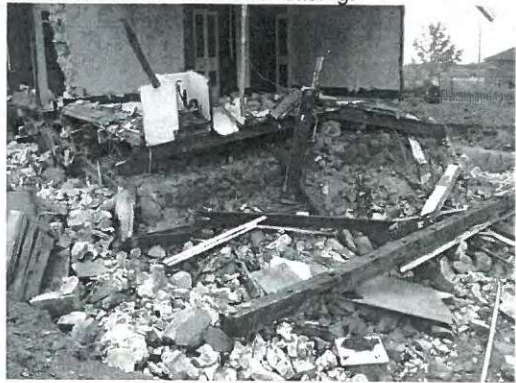
View of southeast corner of salt-box.
