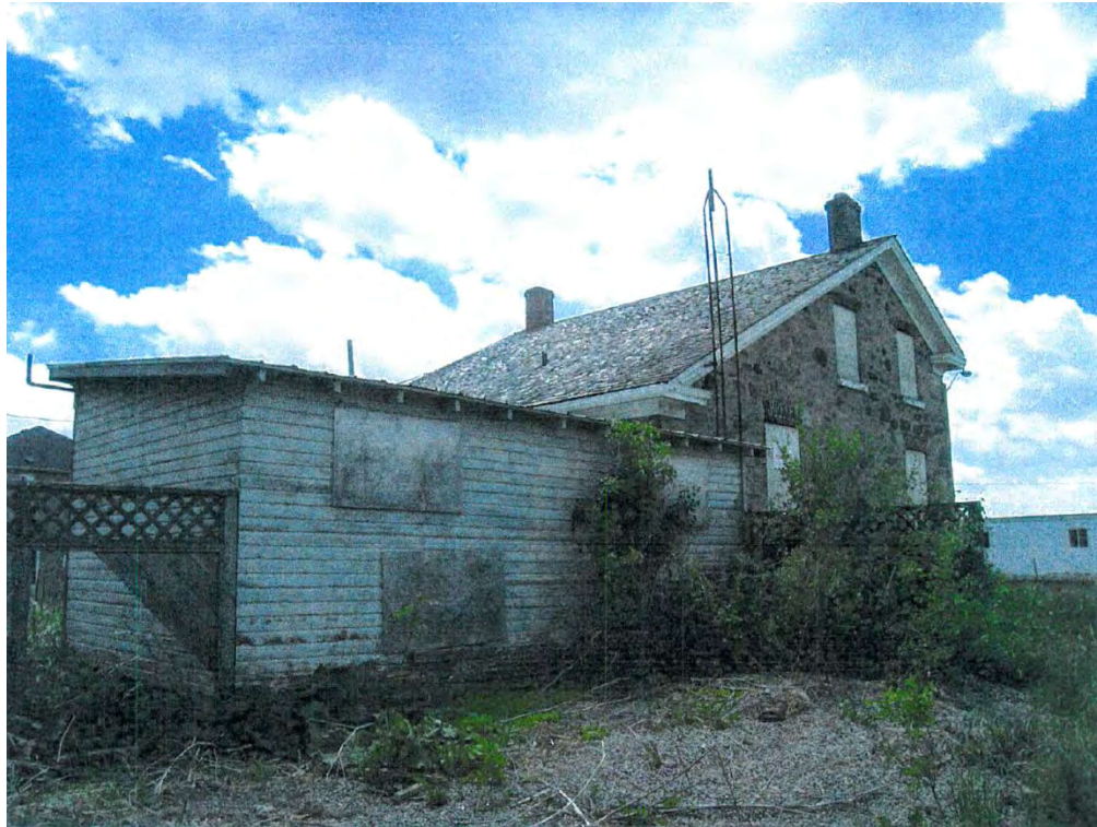
Figure 16: North and east façades of Breadner House prior to demolition (Source: City of Brampton 2009)
