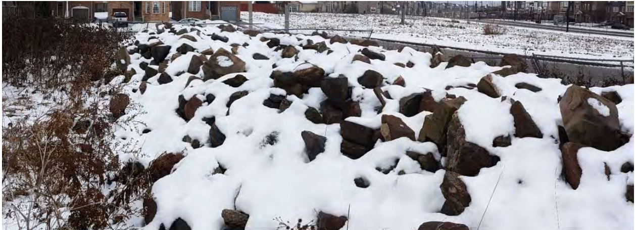
Figure 18: Stones from the collapsed Breadner House on the southeast corner of the original lot (November 2019)
