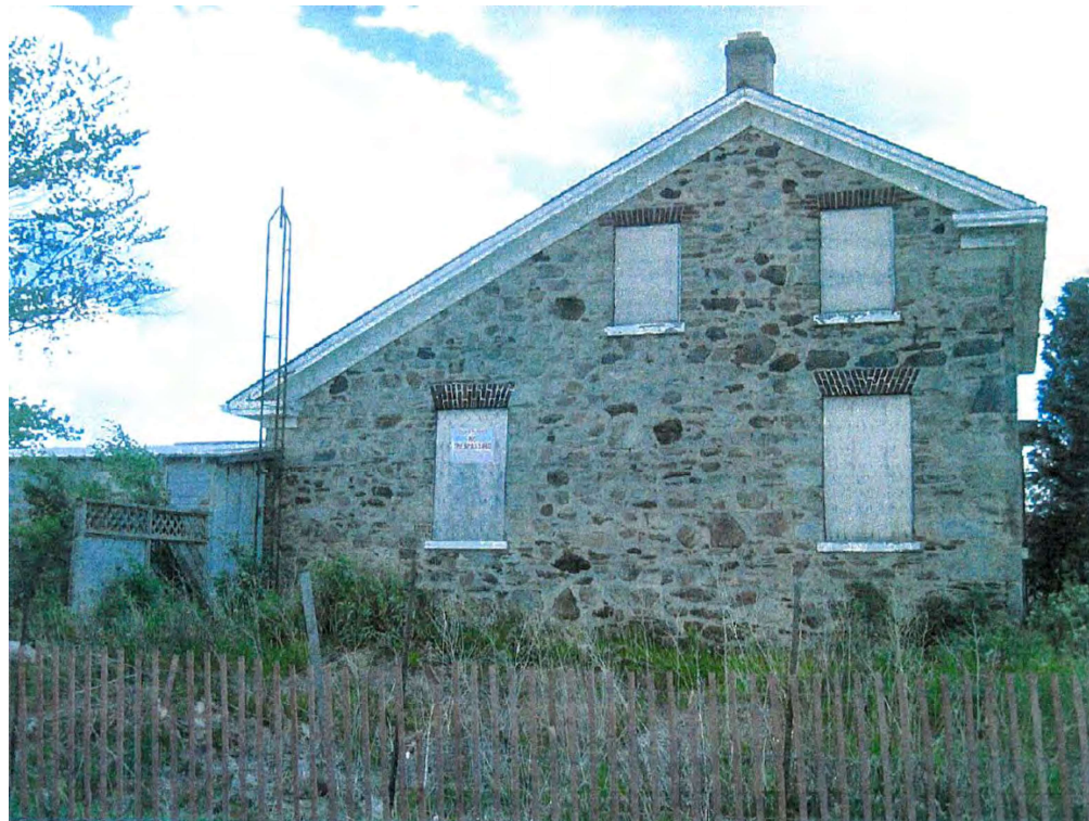
Figure 17: North façade of Breadner House prior to demolition (Source: City of Brampton 2009)
