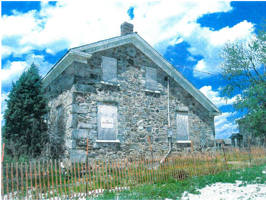
Figure 14: West and south façades of Breadner House prior to demolition (Source: City of Brampton 2009)
