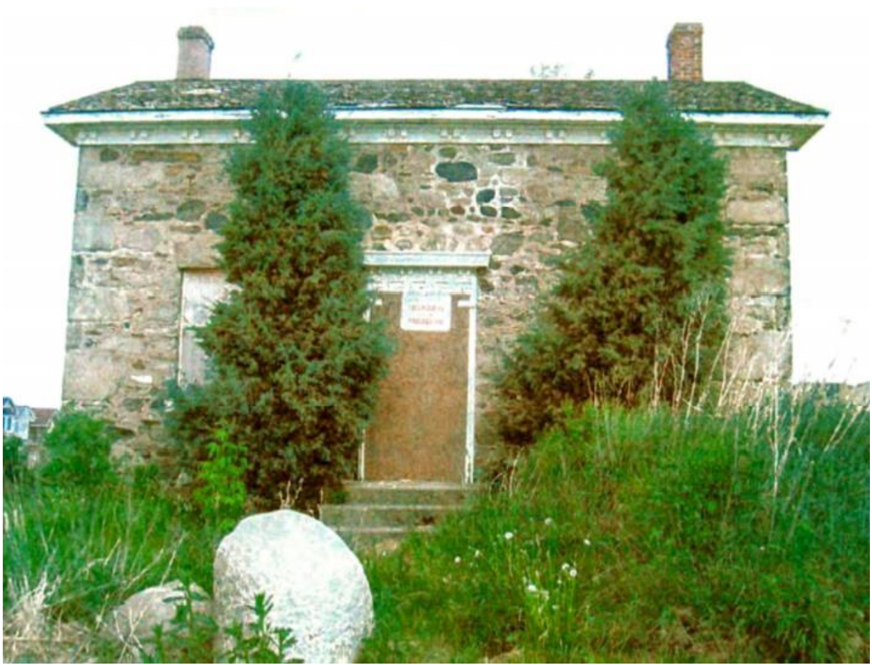
Figure 4: Front (west) elevation of the Breadner House (Source: City of Brampton, 2009)
