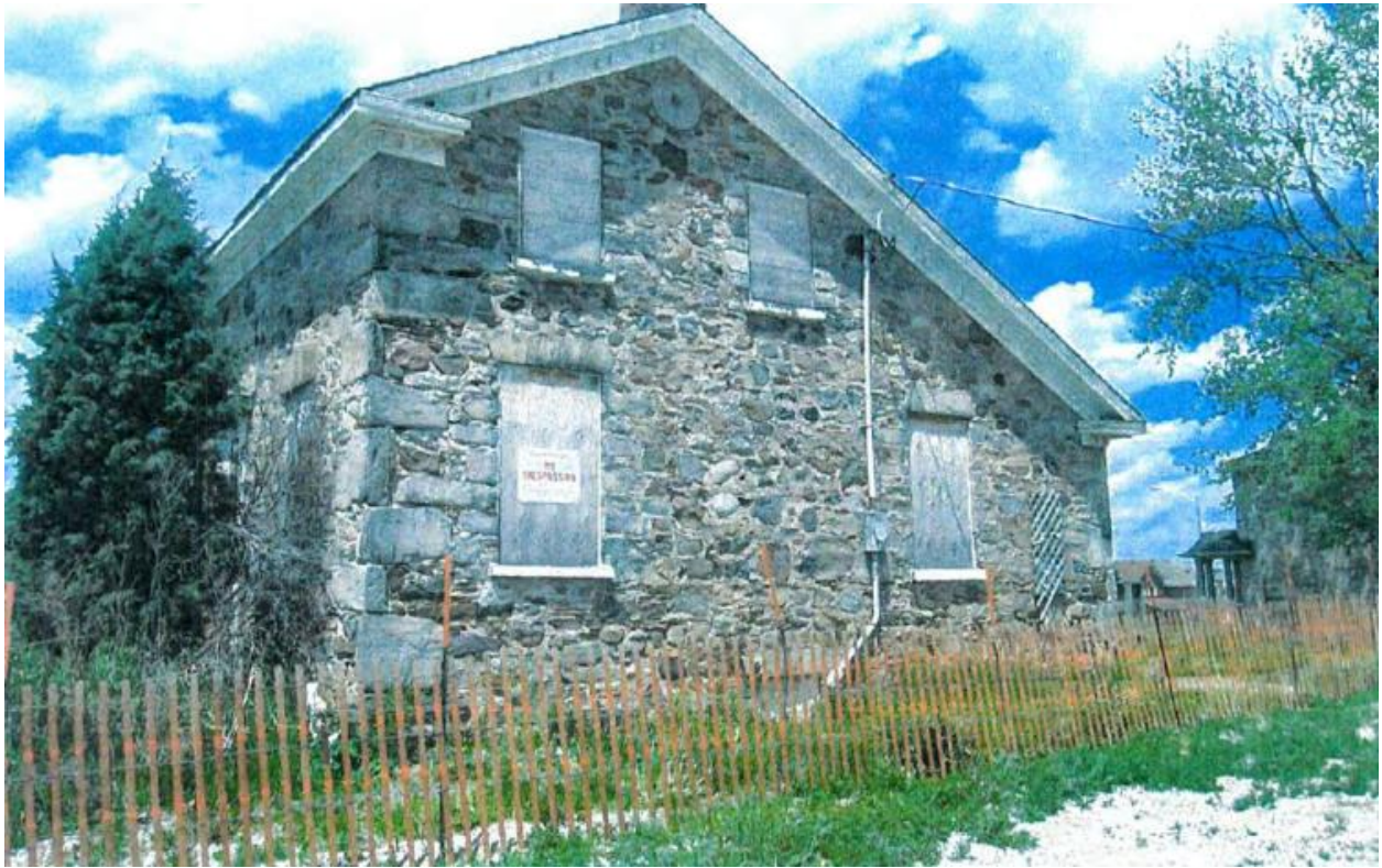
Figure 5: Side (south) elevation of the Breadner House (Source: City of Brampton, 2009)
