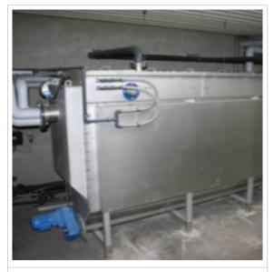
Figure D11.2- Waste Water Source Heat Pump
