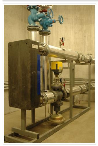
Figure D12.1- Example of District Heating Substation
