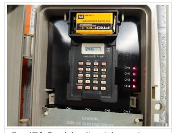
Figure A03.3 – Timerclock used to control some washroom lighting, set to operated 24/7.
