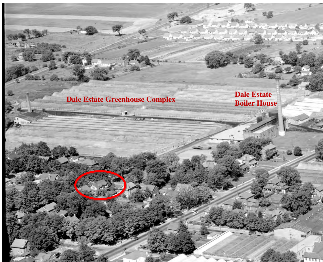
The subject property at 38 Isabella Street (circled) as seen in a circa 1950 aerial photograph of Main Street North and Dale Estate. The photograph helps to illustrate the historical context.
