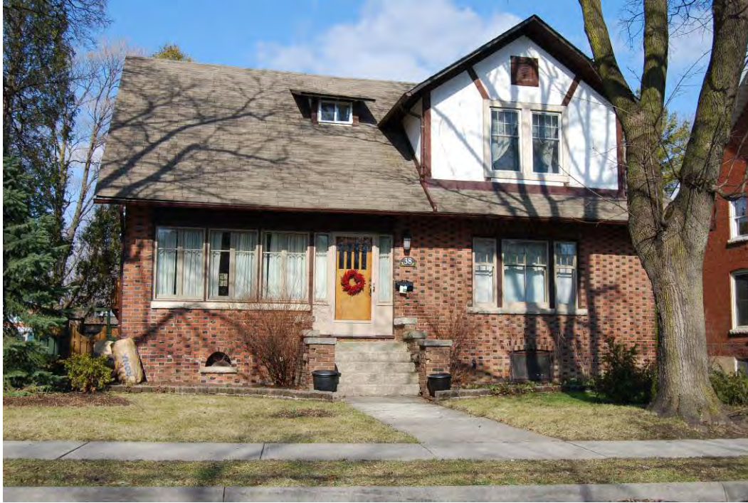
Figure 1: Front elevation of 38 Isabella Street showing textured brick patterning, prominent gabled dormer and small shed dormer, main entrance and other details..
