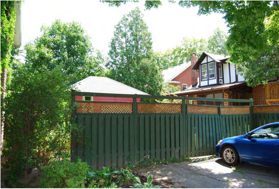
Figure 11: This photo shows portions of the side and rear of the subject property, including the hip roof of the garage, boxed dormer, more half timbering and an enclosed porch at the rear of the house.
