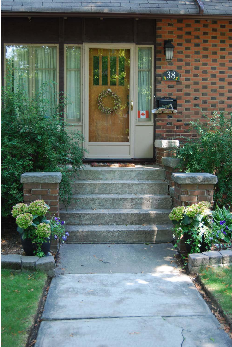
Figure 9: Detail showing front entrance characteristics including masonry knee walls with stone caps that flank the steps, single-leaf oak door with side lights.
