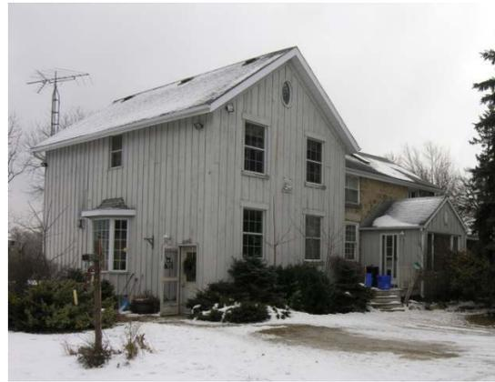
Figure 27 Farmhouse Exterior, view of east and north façades, December 2009, showing the 1991 2-storey addition with board-and-batten cladding also applied to the enclosed porch from 1969.
