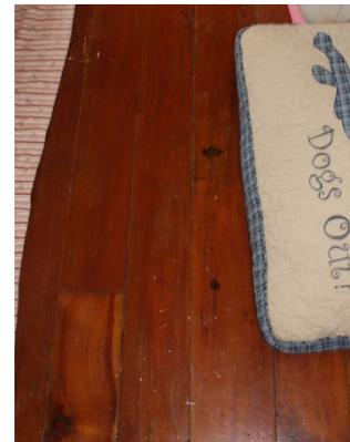
Figure 25 Farmhouse Interior, detail view showing original pine wood plank flooring.
