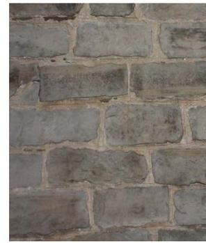
Figure 18: Farmhouse Exterior, detail view of north facade, showing the rough coursed limestone masonry
