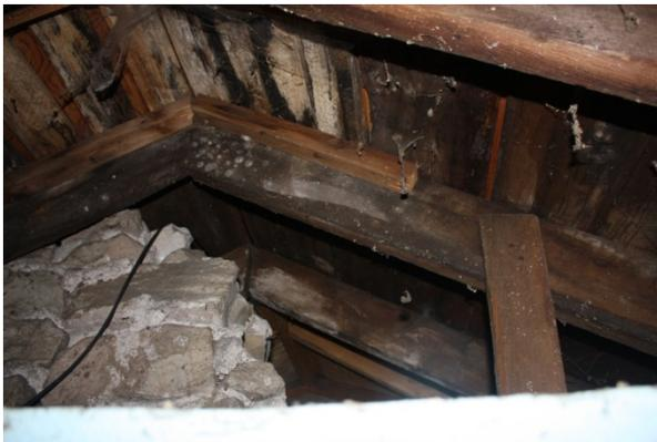
Figure 24 Farmhouse Interior, detail view of the attic showing original hewn roof rafters and decking board
