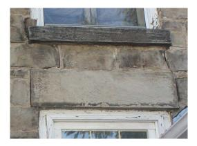
Figure 19 Farmhouse Exterior, detail view of north facade, showing the dressed stone lintels and sills
