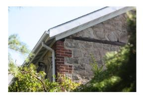
Figure 17: Farmhouse Exterior, detail view of west facade, showing the brick quoins and the horizontal nailer beam from the former porch.
