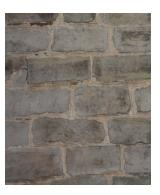
Figure 18: Farmhouse Exterior, detail view of north facade, showing the rough coursed limestone masonry
