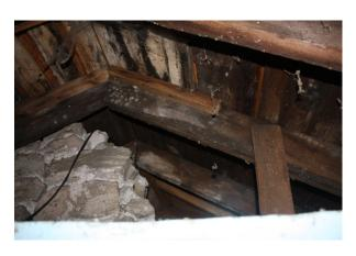
Figure 24 Farmhouse Interior, detail view of the attic showing original hewn roof rafters and decking board (December 2009)
