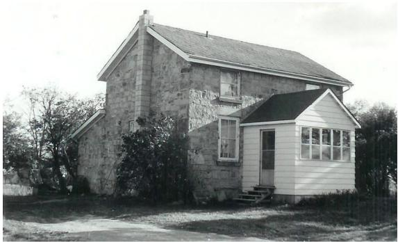
Figure 14: Farmhouse Exterior, view of east and north façades, 11687 Chinguacousy Road, Brampton, c. 1969, showing the wood porch on the north which replaced the original stone summer kitchen and a drive shed and the non-original concrete block chimney on the east.
