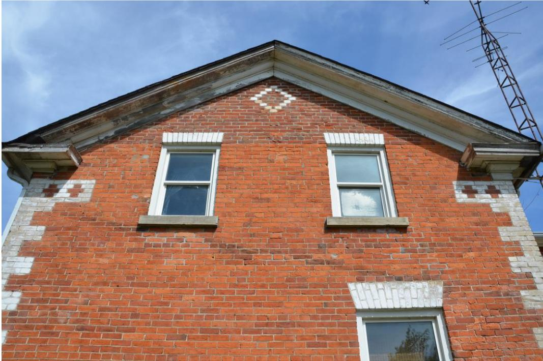
Figure 4: Image of the south façade of the Farmhouse exhibiting wood cornice, eaves, and eave returns; dichromatic brickwork and stringcourse; and fenestration of gable ends (Source: City of Brampton, 2018).
