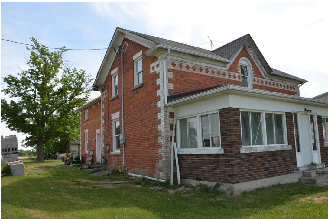
Figure 5: View of the front (west) façade and north façade of the Farmhouse, showing the front section and the rear wing. The dichromatic brickwork, central gable with arched window, and cross gable roof are visible (Source: City of Brampton, 2018).
