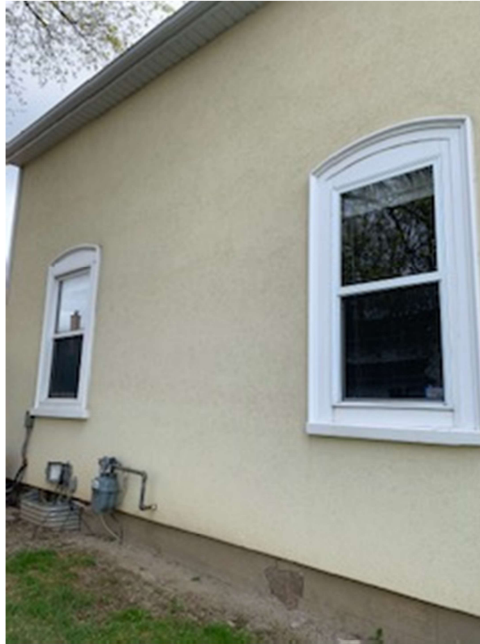
North Side, Vinyl Window in Front, Wood Window at Back
