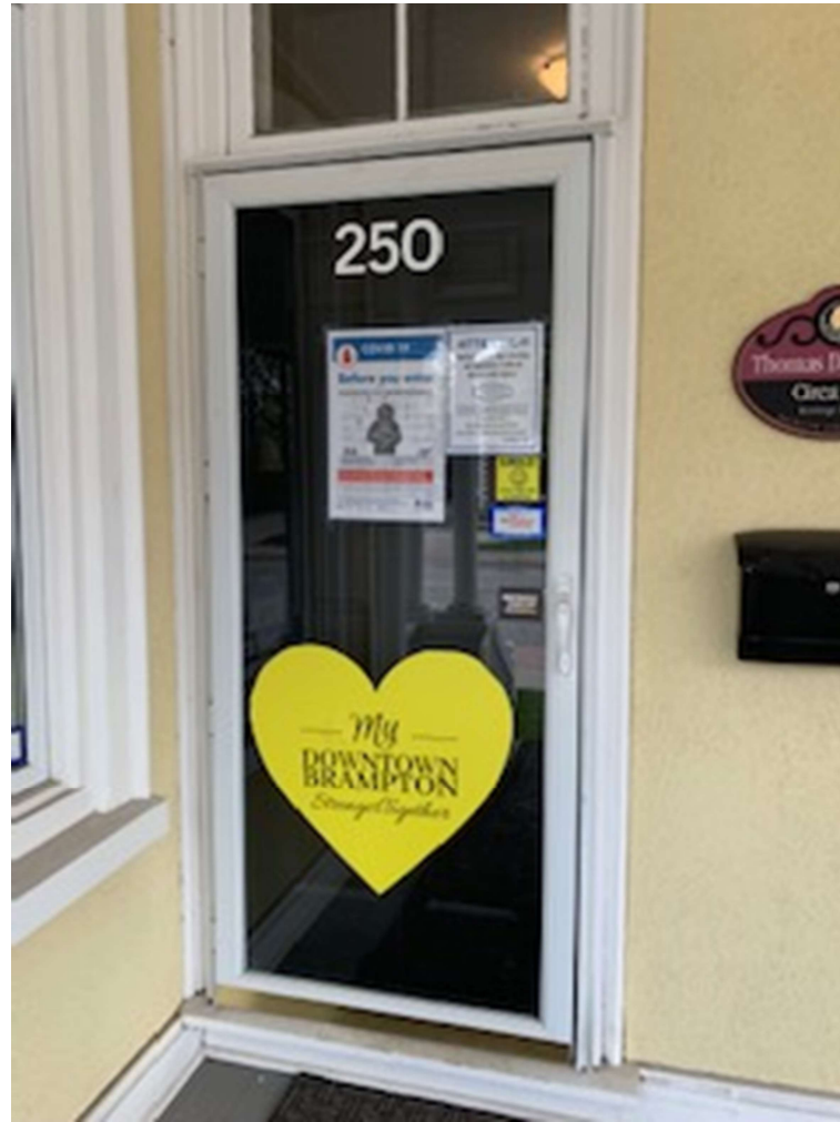
Existing Front Door with Metal Storm Door
