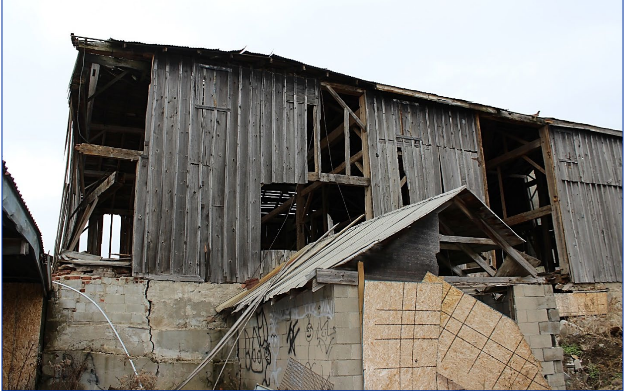
Figure 10: Southwest corner (Source: LHC, December 2020).
