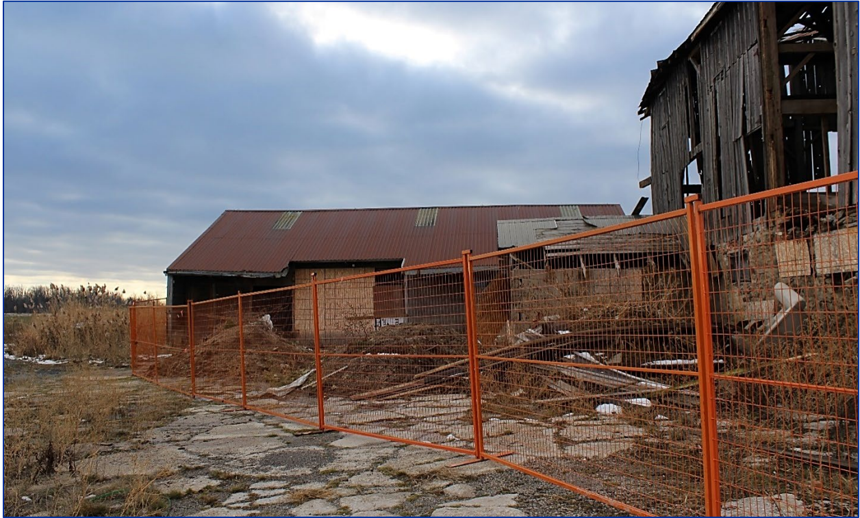
Figure 18: Eastern elevation (Source: LHC, December 2020).
