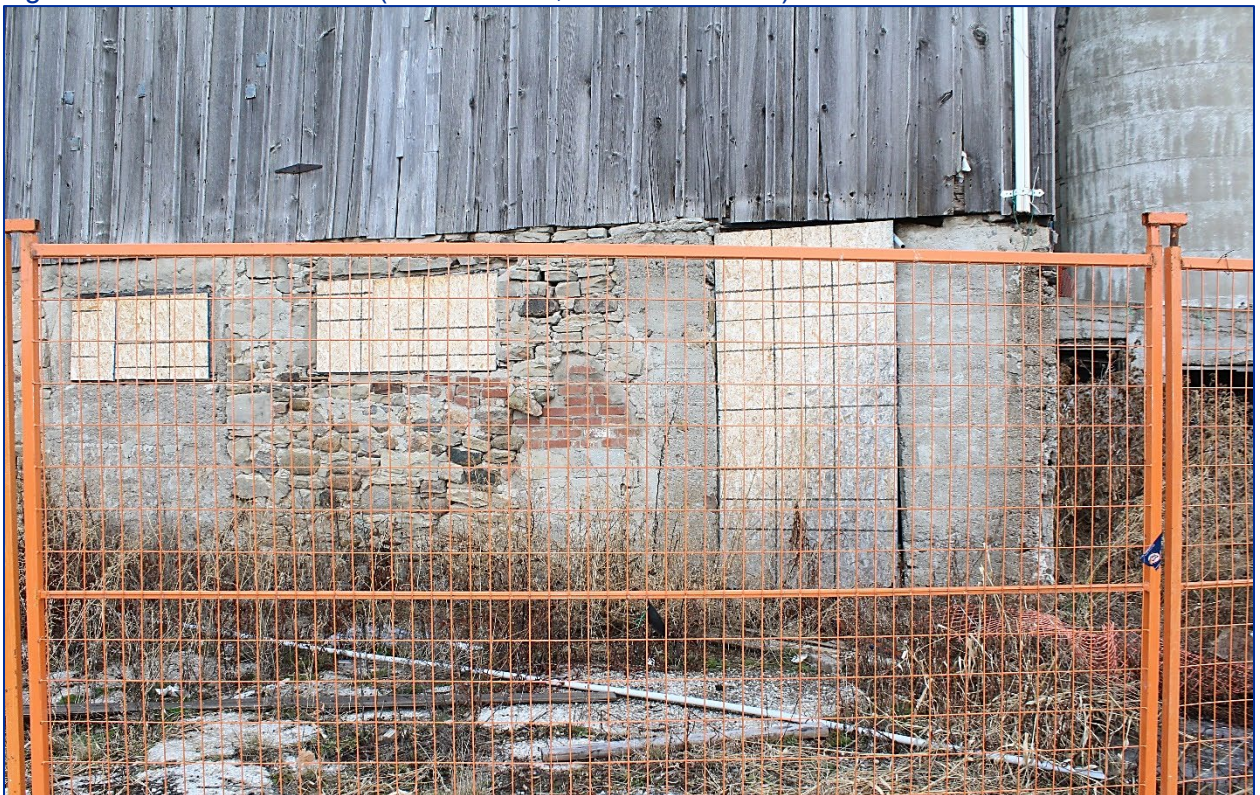
Figure 9: Southeast elevation foundation (Source: LHC, December 2020).
