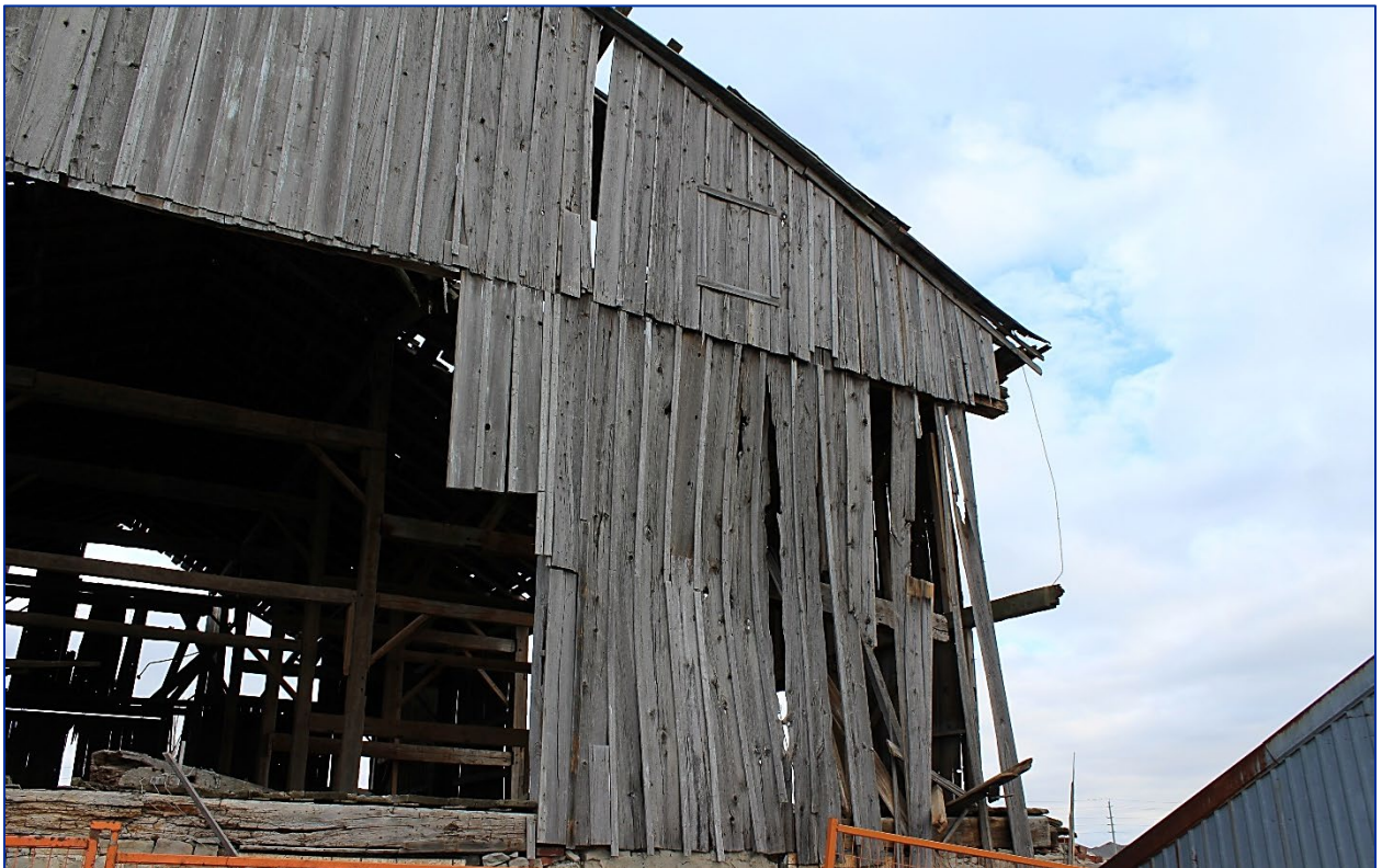
Figure 13: Southwest corner (Source: LHC, December 2020).
