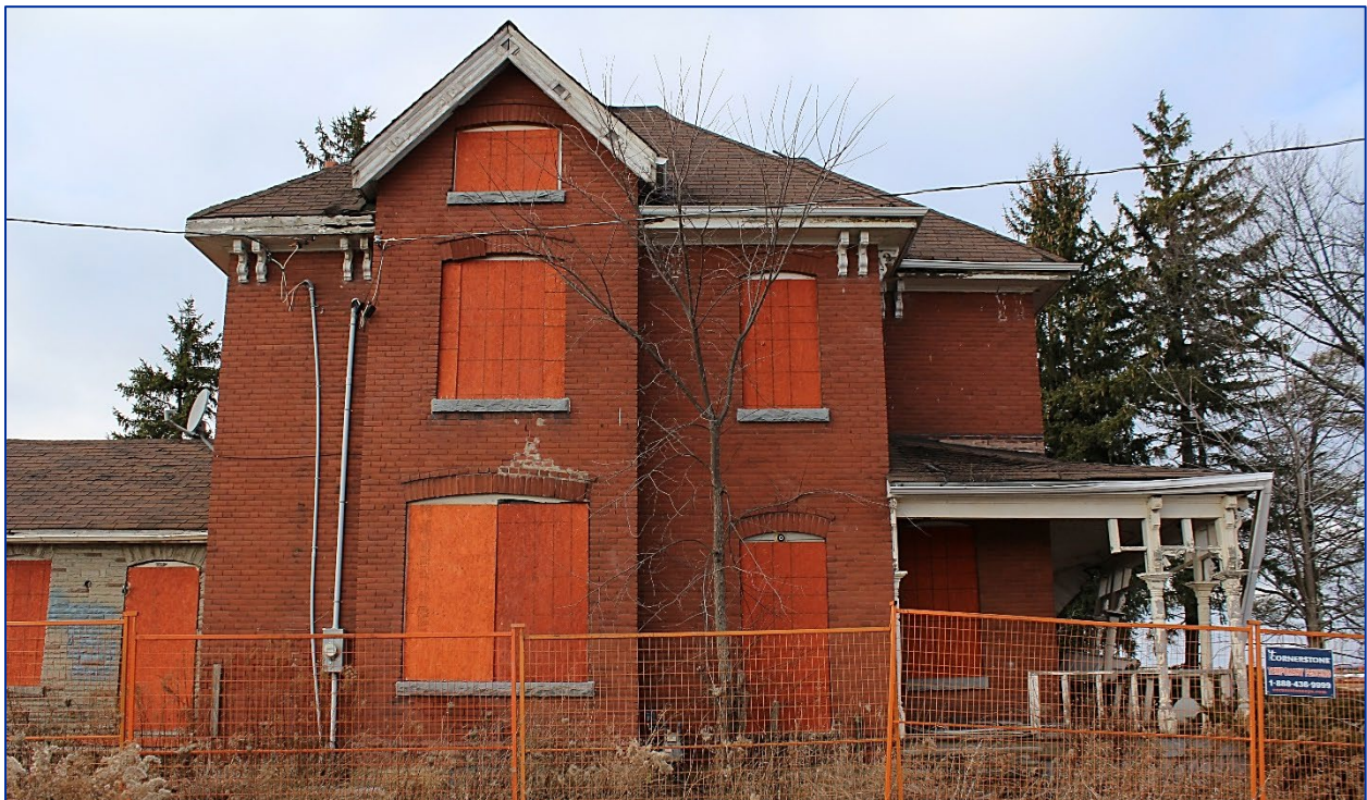
Figure 3: Southern elevation (Source: LHC, December 2020).
