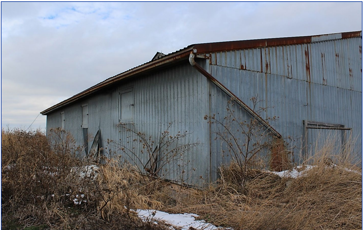
Figure 21: Southwest elevation (Source: LHC, December 2020).
