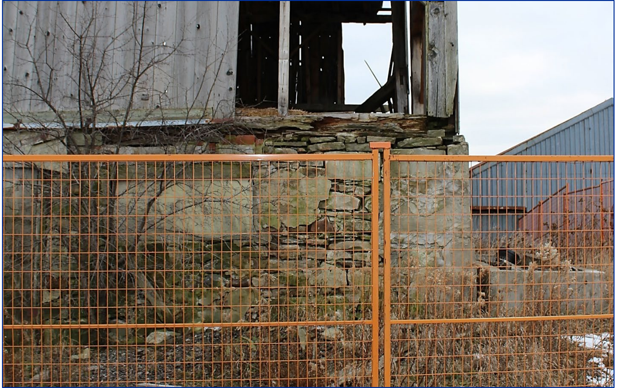
Figure 16: Northwest corner foundation (Source: LHC, December 2020).
