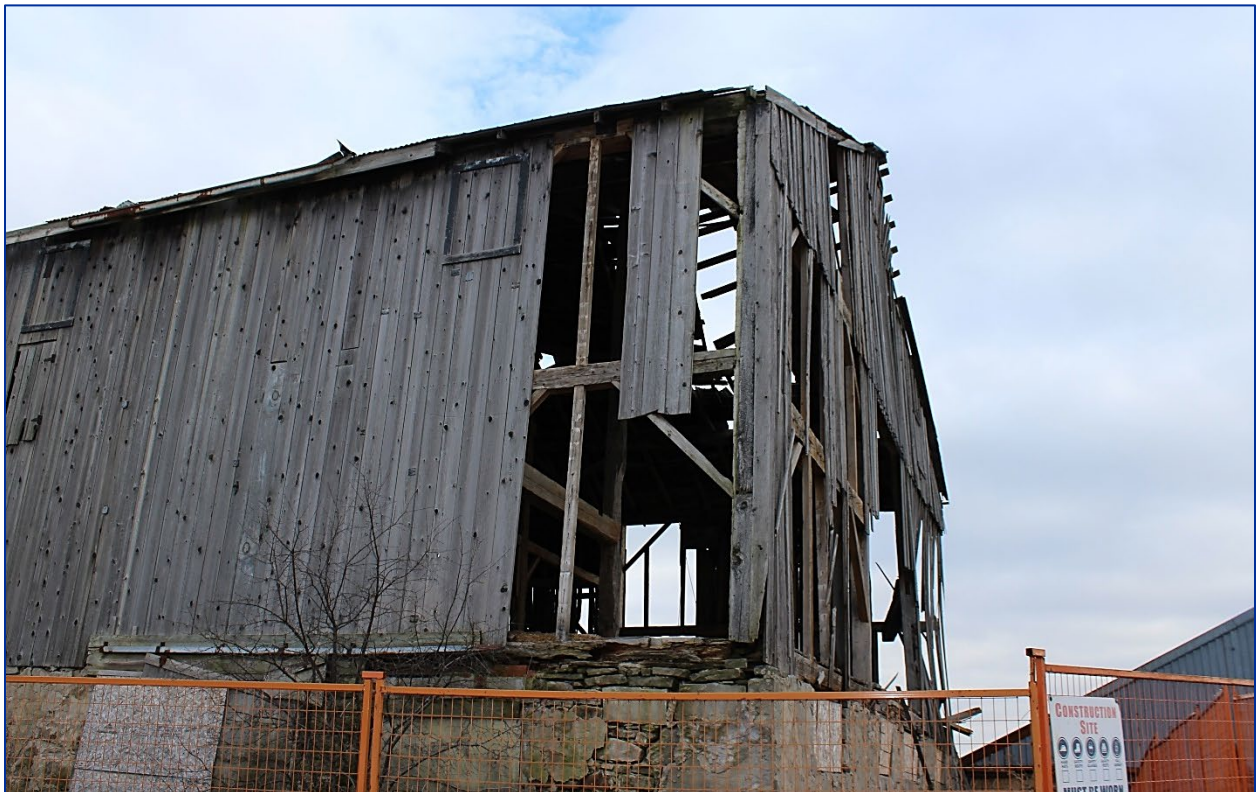
Figure 15: Northern elevation (Source: LHC, December 2020).
