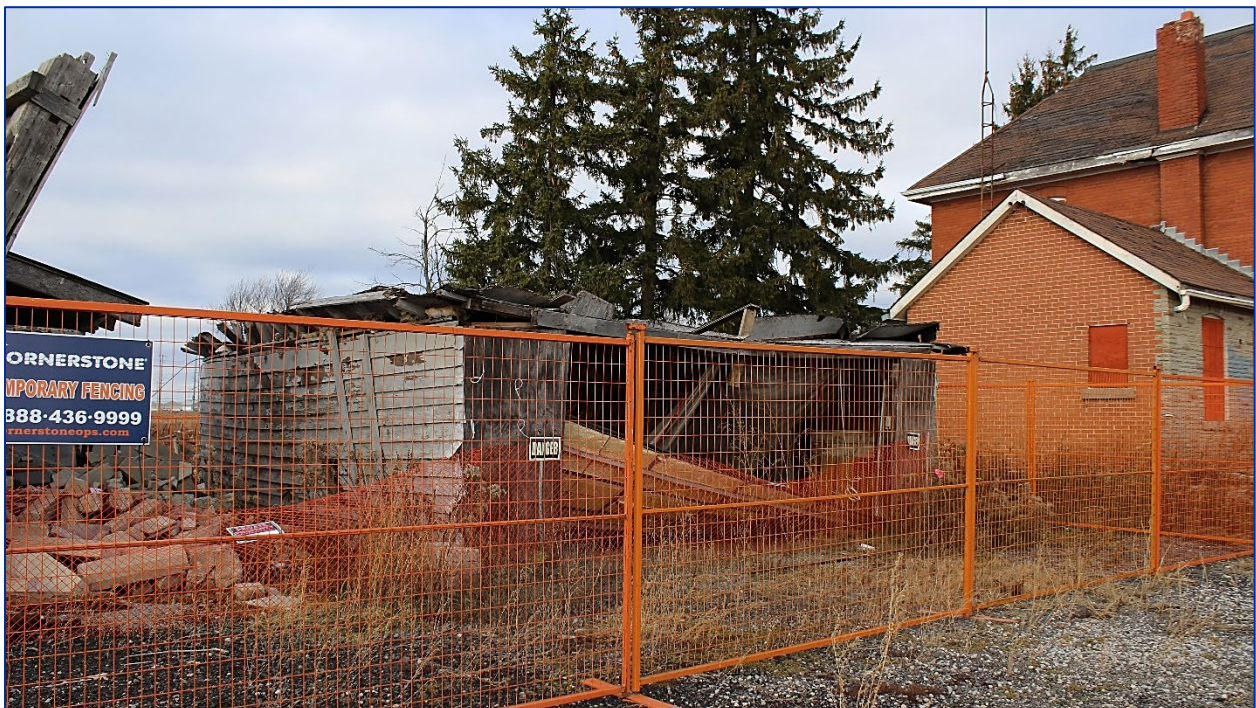
Figure 28: Southwestern corner (Source: LHC, December 2020).
