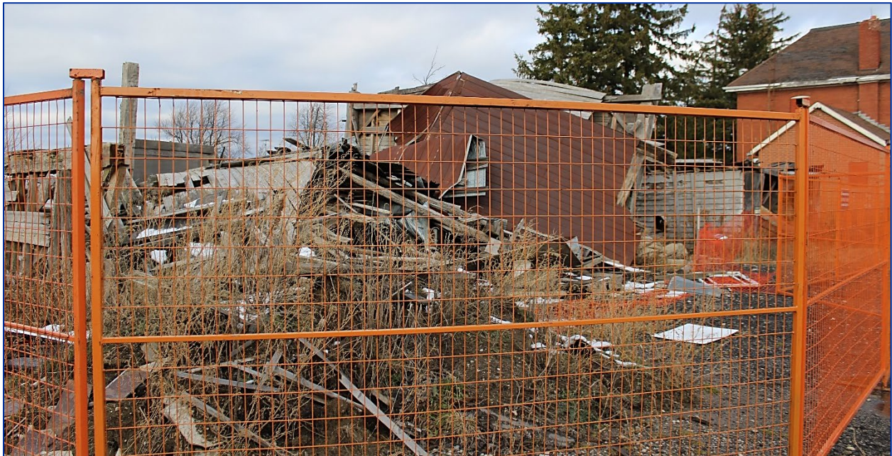
Figure 30: Southwestern corner (Source: LHC, December 2020).
