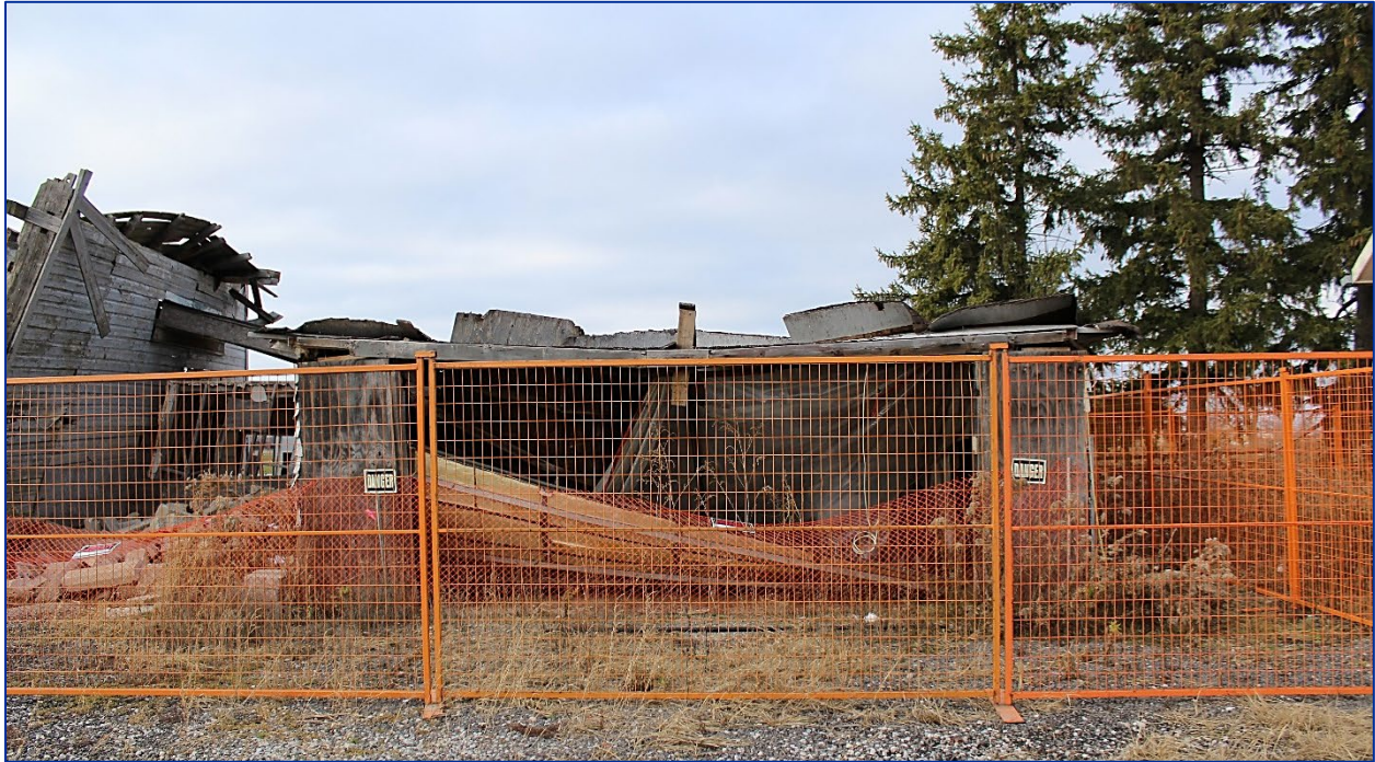
Figure 27: Southern elevation (Source: LHC, December 2020).
