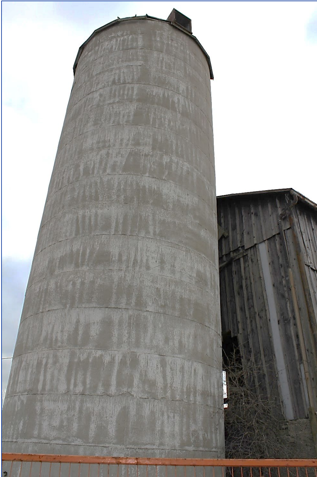
Figure 17: Northern elevation (Source: LHC, December 2020).
