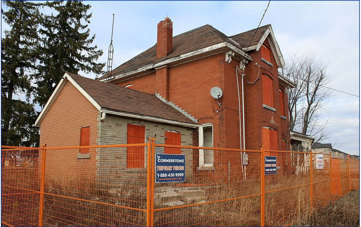
Figure 4: Southwest elevation (Source: LHC, December 2020).
