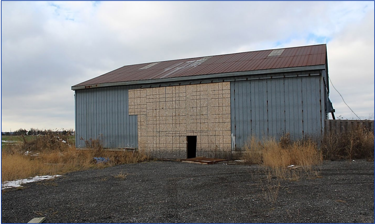
Figure 23: Southern elevation (Source: LHC, December 2020).
