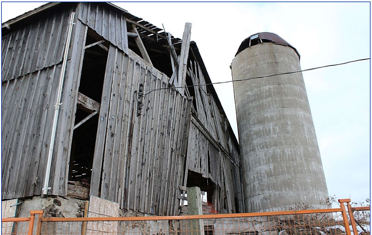
Figure 7: Eastern elevation detail (Source: LHC, December 2020).
