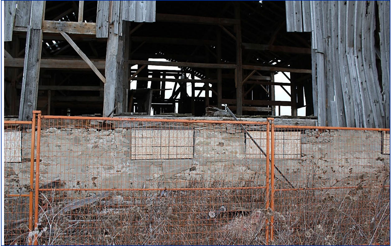
Figure 12: Western elevation foundation (Source: LHC, December 2020).
