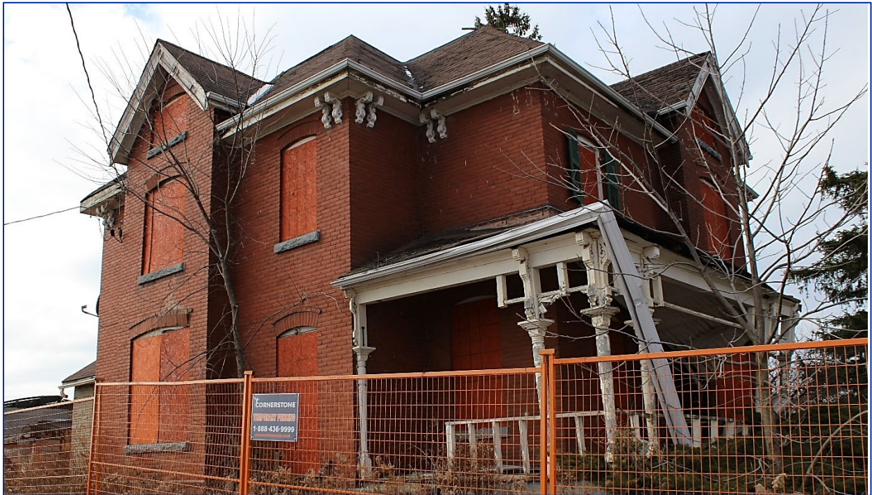
Figure 2: Southeast elevation (Source: LHC, December 2020).
