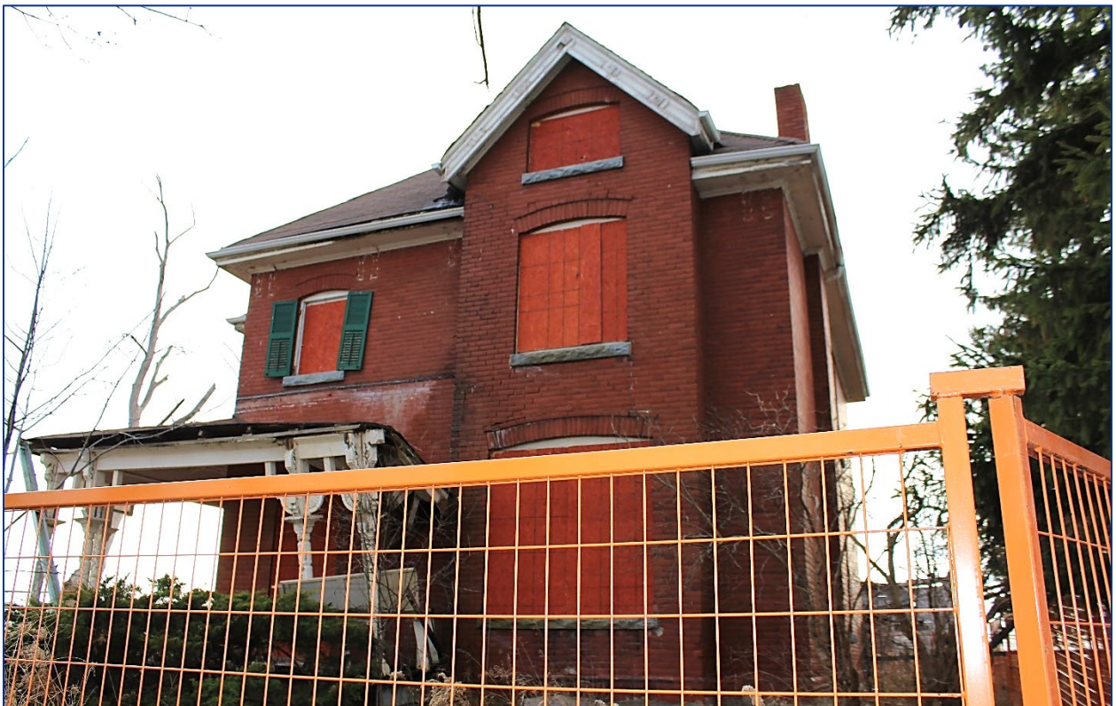
Figure 5: Eastern elevation (Source: LHC, December 2020).
