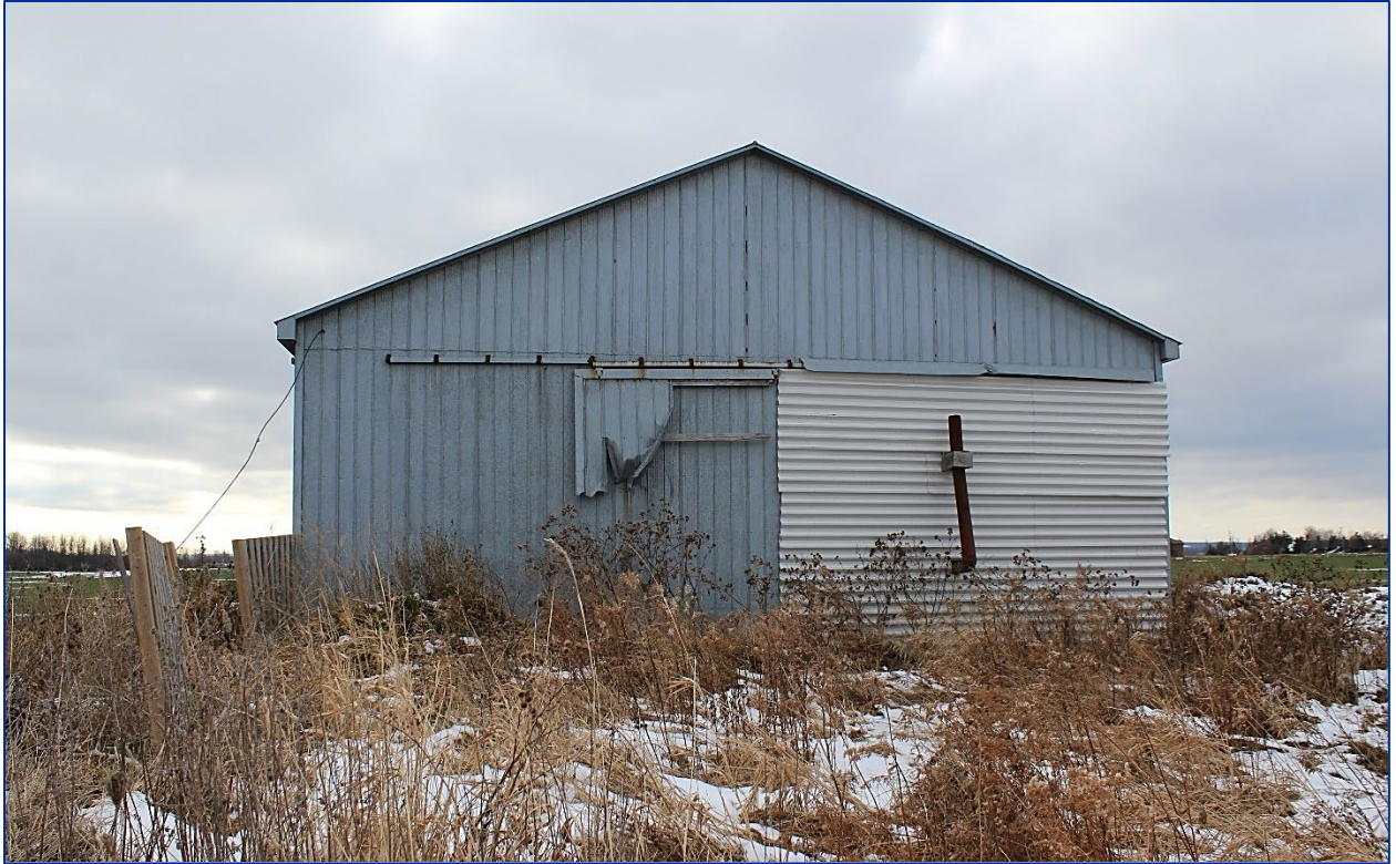
Figure 25: Eastern elevation (Source: LHC, December 2020).
