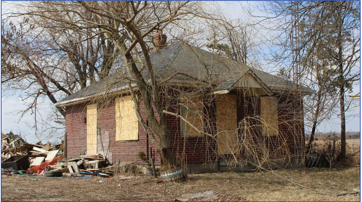
Figure 31: Southwestern elevation (Source: LHC, December 2020).
