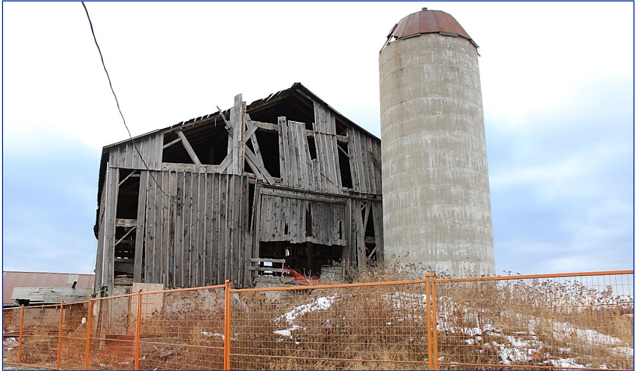
Figure 6: Eastern elevation (Source: LHC, December 2020).
