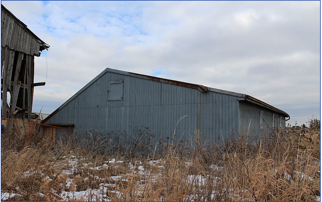
Figure 20: Northern elevation (Source: LHC, December 2020).
