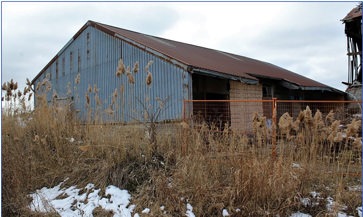
Figure 19: Southeast corner (Source: LHC, December 2020).
