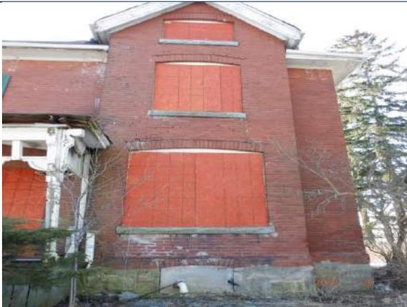
*Figure 4.2.2: Mortar joint deterioration below hoarding at window openings at east wall of Farmhouse.*
