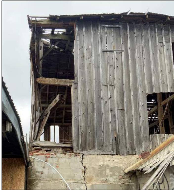
**Photograph 3: Damaged south endwall frame**
