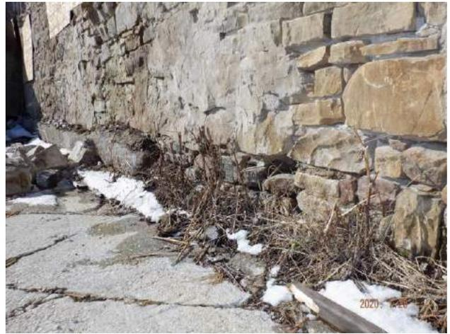
Figure 4.2.36: Typical example of deteriorated mortar at base of rubble stone foundation wall.
