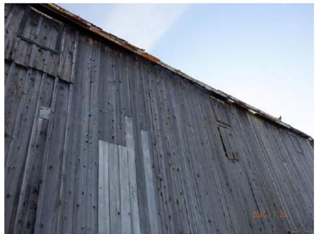
Figure 4.2.41: Missing eavestrough at top of north wall. Sections of eavestrough were found lying on the ground below.
