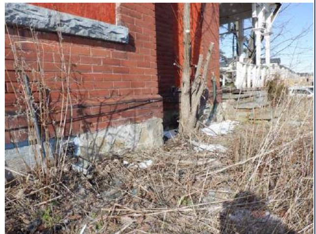
*Figure 4.2.12: Deteriorated mortar joints at base of south wall.*
