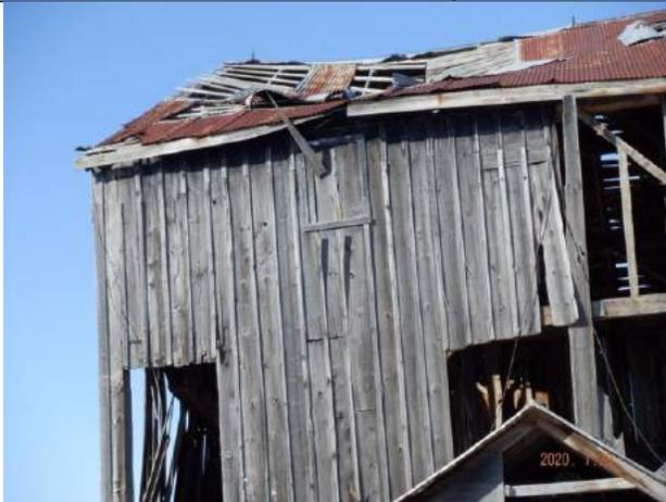
Figure 4.2.33: Roof collapse at west end of roof
