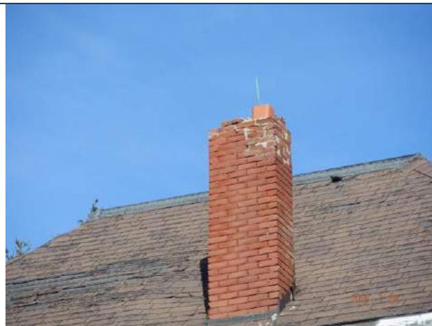
Figure 4.2.14: Deteriorated brick masonry and missing cap at chimney on west side of Farmhouse roof. Also note deteriorated asphalt shingles.
