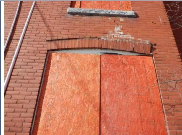
*Figure 4.2.9: Deteriorated bricks and mortar at arch over first storey window in south wall. Schedule B of the Order refers to the bricks forming the arch as “radiating voussoirs” that contribute to the heritage value of the Farmhouse.*
