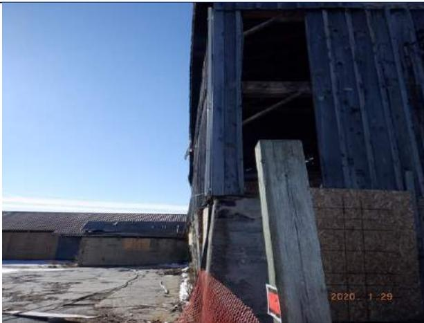
Figure 4.2.37: Outward movement at top of south foundation wall
