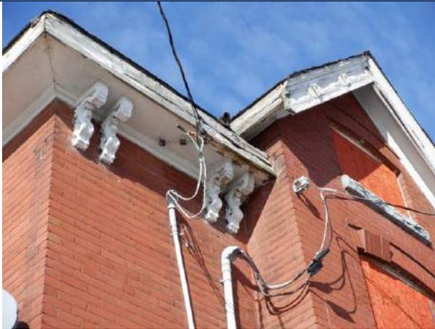
Figure 4.2.7: Deteriorated soffit and fascia at south wall
