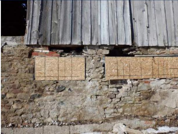
Figure 4.2.35: Large sections of missing rubble stone at south foundation wall.
