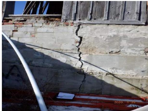
Figure 4.2.34: Large crack in foundation at southwest corner
