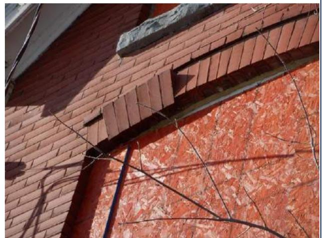
*Figure 4.2.10: Dislodged bricks at arch over second storey window in south wall are in danger of falling.*
