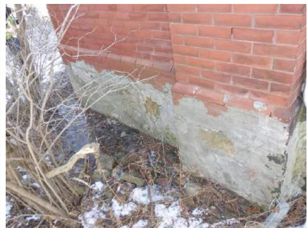
Figure 4.2.21: Deteriorated mortar joints at base of north wall of Farmhouse.
