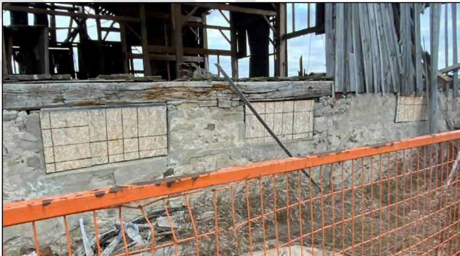
**Photograph 6: Deteriorated sill plate, south endwall**
