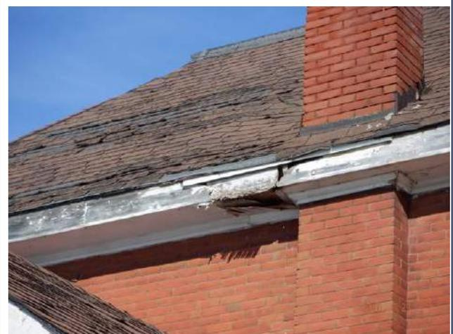
Figure 4.2.15: Deteriorated asphalt shingles, soffit and fascia at west side of Farmhouse.
