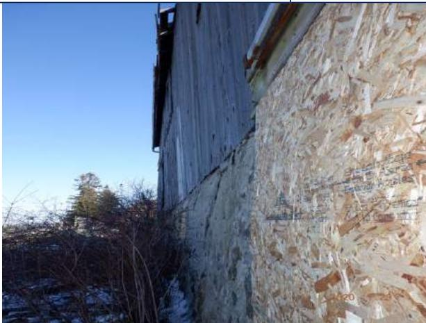
Figure 4.2.40: Significant inward movement at top of north foundation wall. The wall is at risk of instability and collapse.
