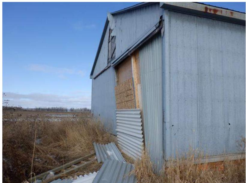
Figure 4.2.27: Impact damage at west wall of Drive Shed
