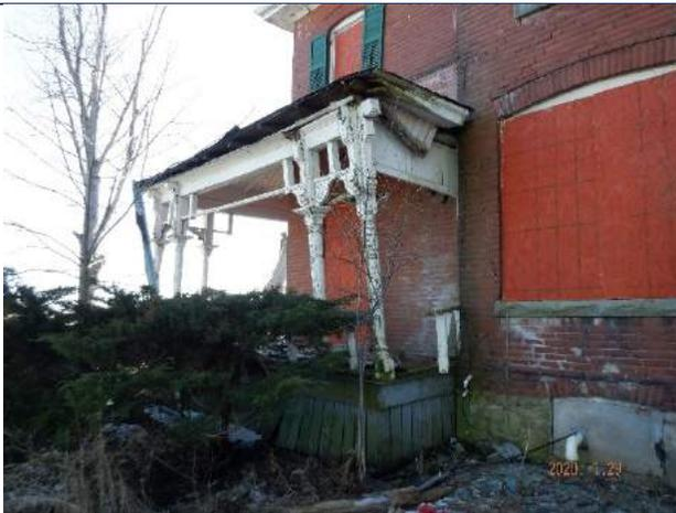
*Figure 4.2.4: Deteriorated wraparound porch at east wall with ornamental turned wood posts. Posts are structurally unstable.*
