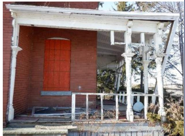
*Figure 4.2.5: Deteriorated wraparound porch at south wall with ornamental turned wood posts. Posts are structurally unstable. Eavestrough has collapsed.*
