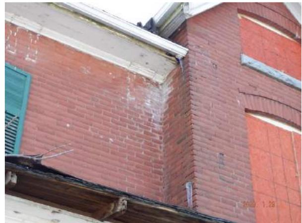
*Figure 4.2.3: Deteriorated soffit and mortar joints at east wall of Farmhouse. Also note missing paired ornamental wood brackets below soffit.*
