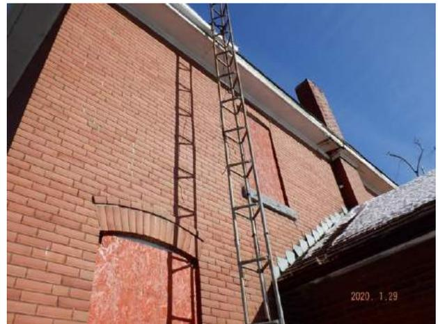
*Figure 4.2.17: Missing section of eavestrough at Farmhouse roof and damaged step flashing where roof of addition meets west wall of Farmhouse.*
