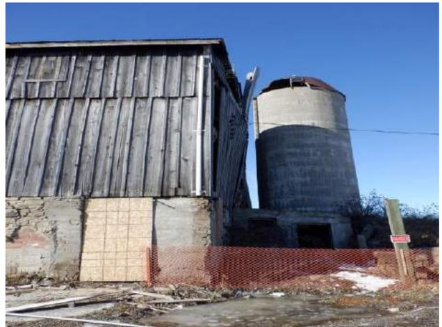
Figure 4.2.38: Missing section of roof at top of concrete silo
