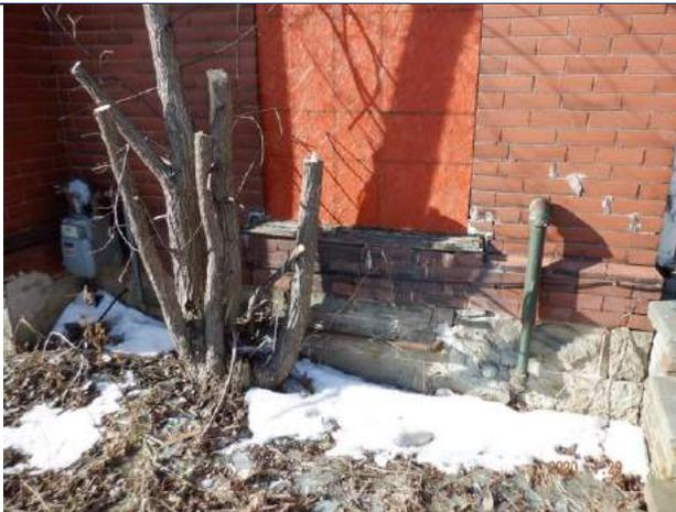
*Figure 4.2.11: Missing stone sill at first storey window in south wall.*
