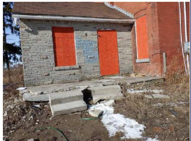
Figure 4.2.8: Deteriorated steps and structural slab over cistern at south side of addition.
