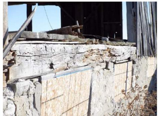
Figure 4.2.44: Rotted timber sill at base of west endwall. The top of this wall is leaning outward.
