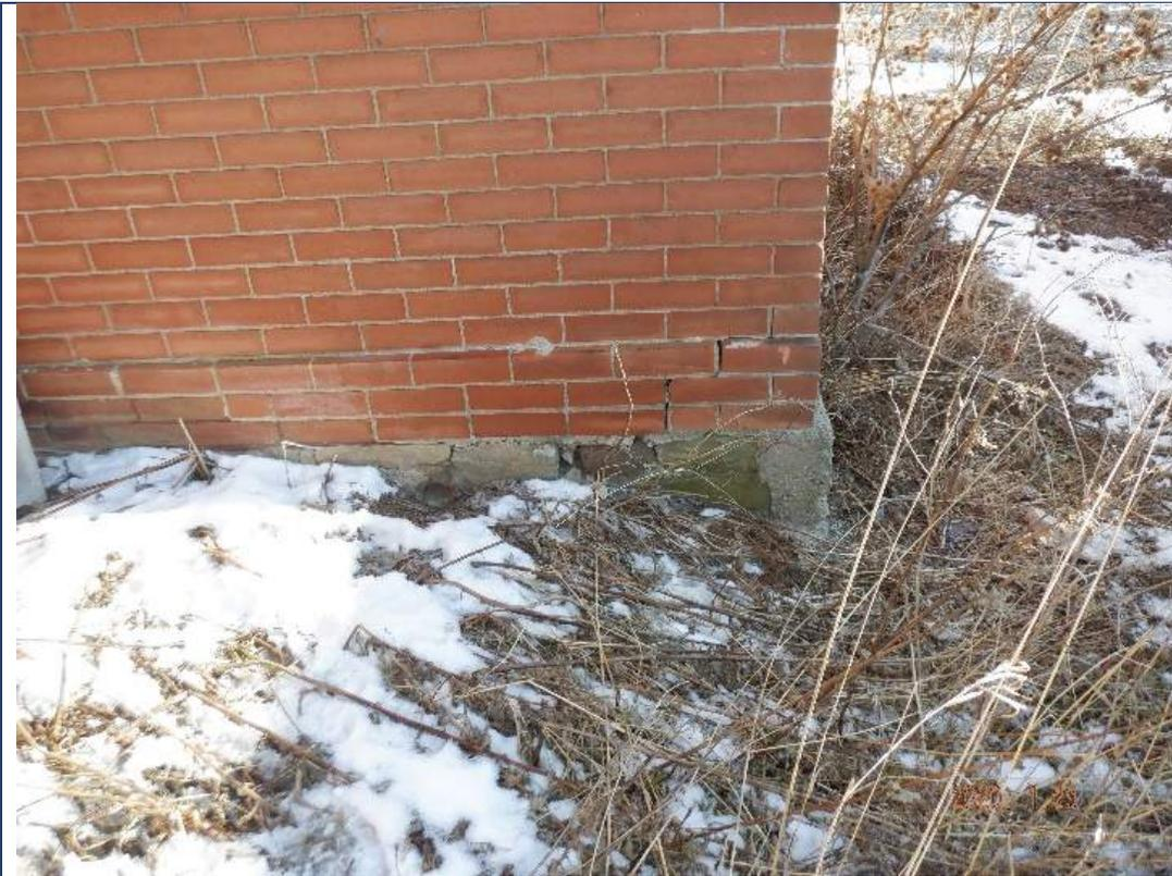
*Figure 4.2.22: Deteriorated mortar joints at base of north wall of Farmhouse addition.*
