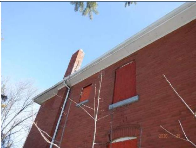
Figure 4.2.20: Defects in north Farmhouse wall include missing brick at arch above lower window, deteriorated masonry between window openings, missing paired ornamental wood brackets below soffit, deteriorated brick masonry at top of chimney and missing chimney cap.
