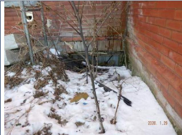
*Figure 4.2.16: Deteriorated brick masonry near grade and deteriorated wood frame of crawl space access hatch at base of west wall of Farmhouse.*
