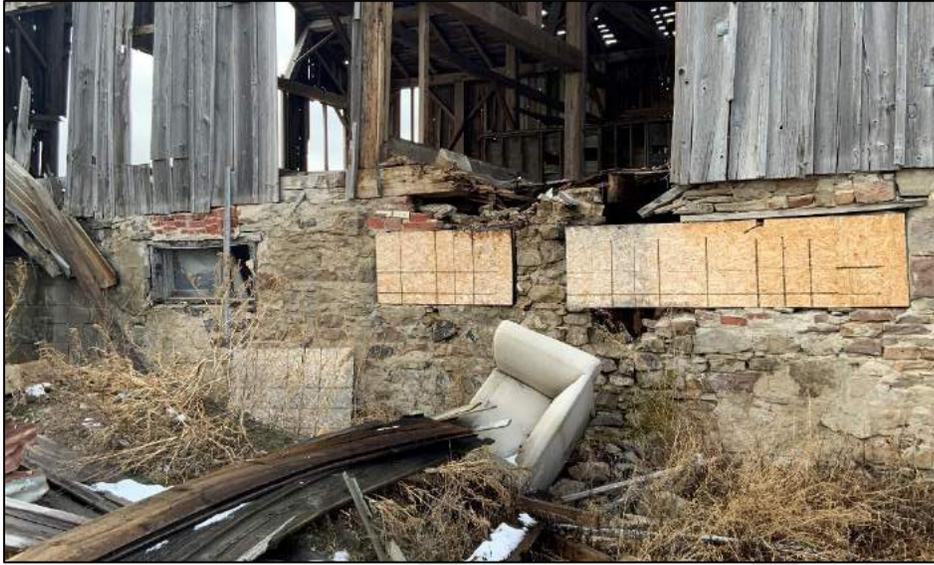
**Photograph 5: Destabilized rubblestone foundation wall**
