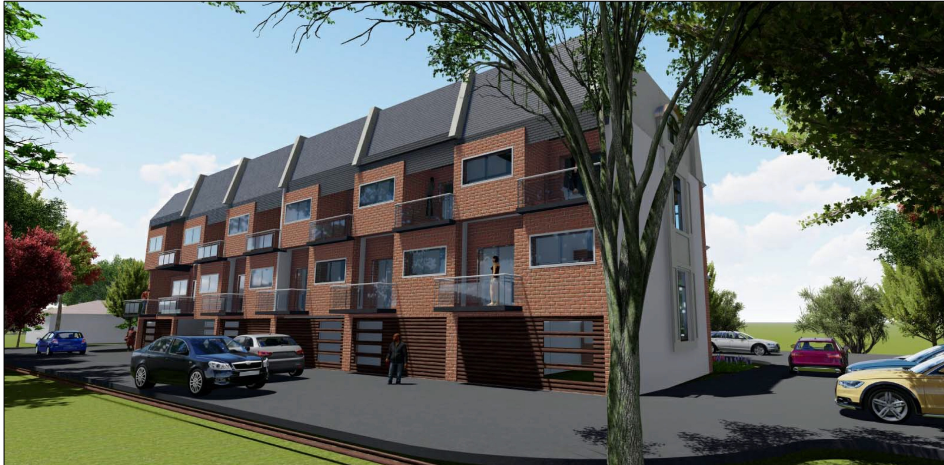
REAR VIEW – GARAGES
